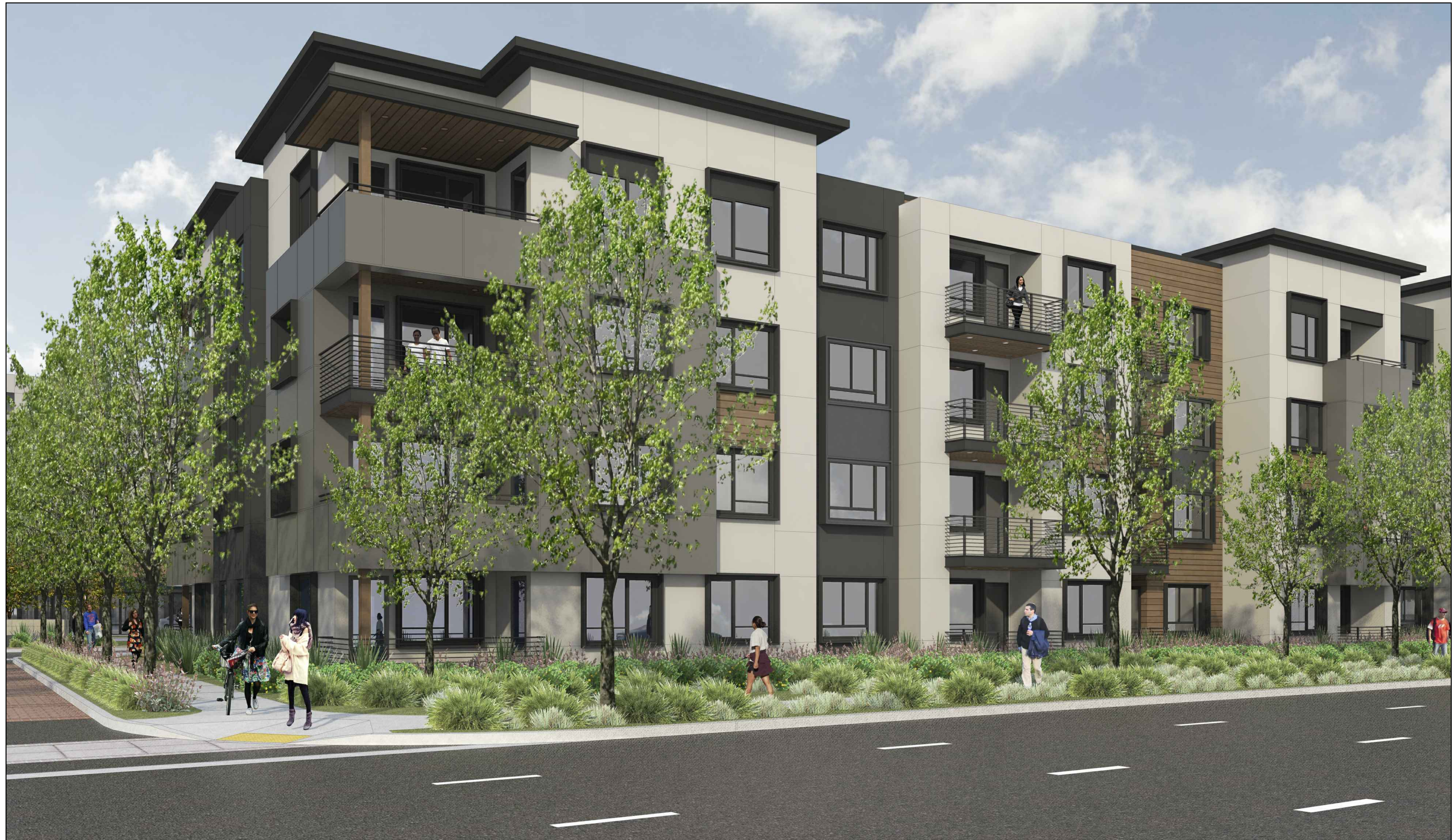
Building A at Entry Drive
