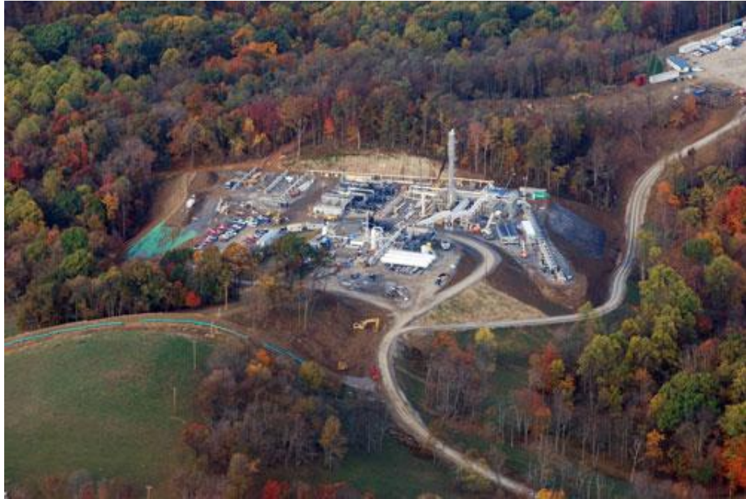
Figure 32: Example of a cryogenic processing facility recently constructed in the Marcellus. This is Caiman Energy's Fort Beeler facility. Processes 'wet' Marcellus gas by cryogenic process removes profitable liquids such as ethane, butane and propane leaving 'dry' methane gas. (from www.marcellus-shale.us/MARCELLUS )
