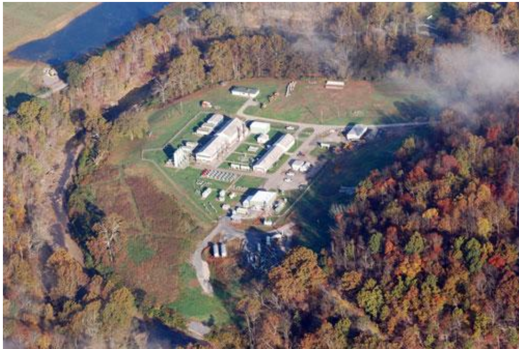
Figure 31: Gas compressor station in the Marcellus. (from www.marcellus-shale.us/MARCELLUS )
