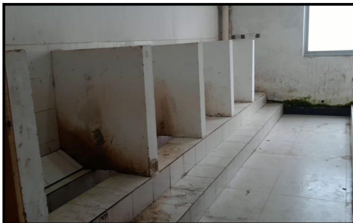
Restroom. There is one on each floor in the dormitories.
