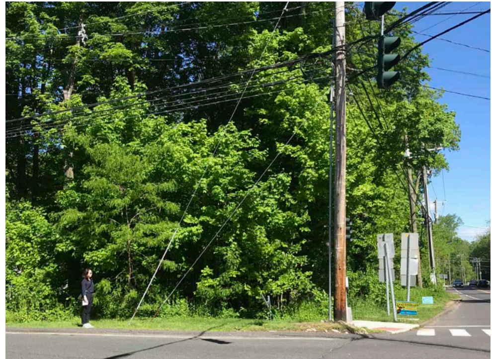
Lack of Sidewalks Leading to Crosswalk
