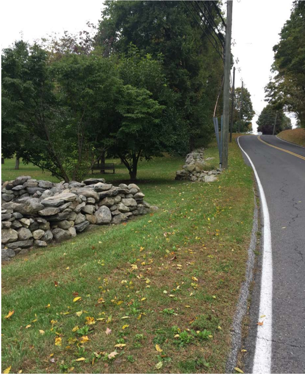
Horizontal & Vertical Road Alignments and a Lack of Roadway Shoulder Limit Safe Bicycle Activity
