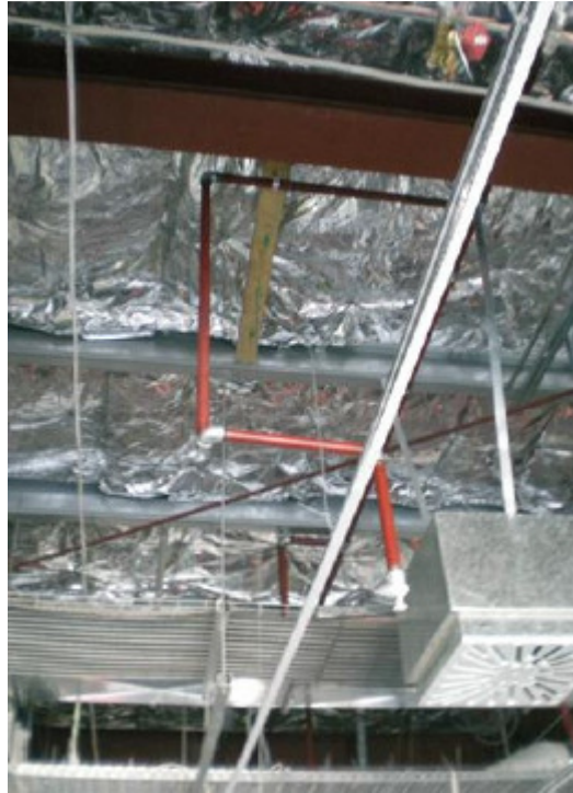
Figure 7: Unrestrained diffusers
