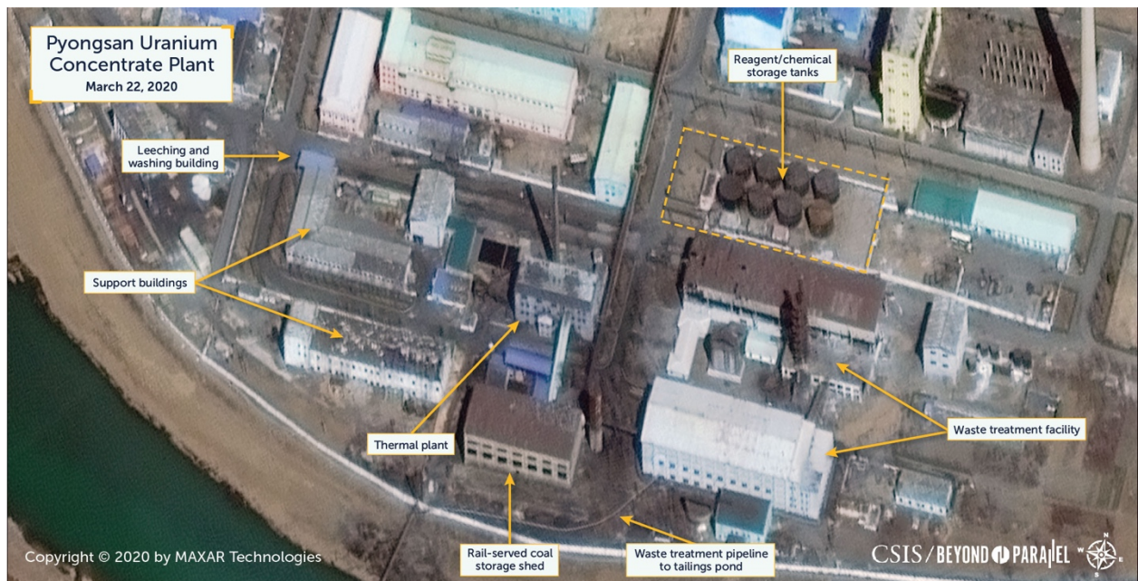
Overview of the southern section of the Pyongsan Uranium Concentrate Plant as of March 22, 2020. (Copyright © 2020 by Maxar Technologies)
