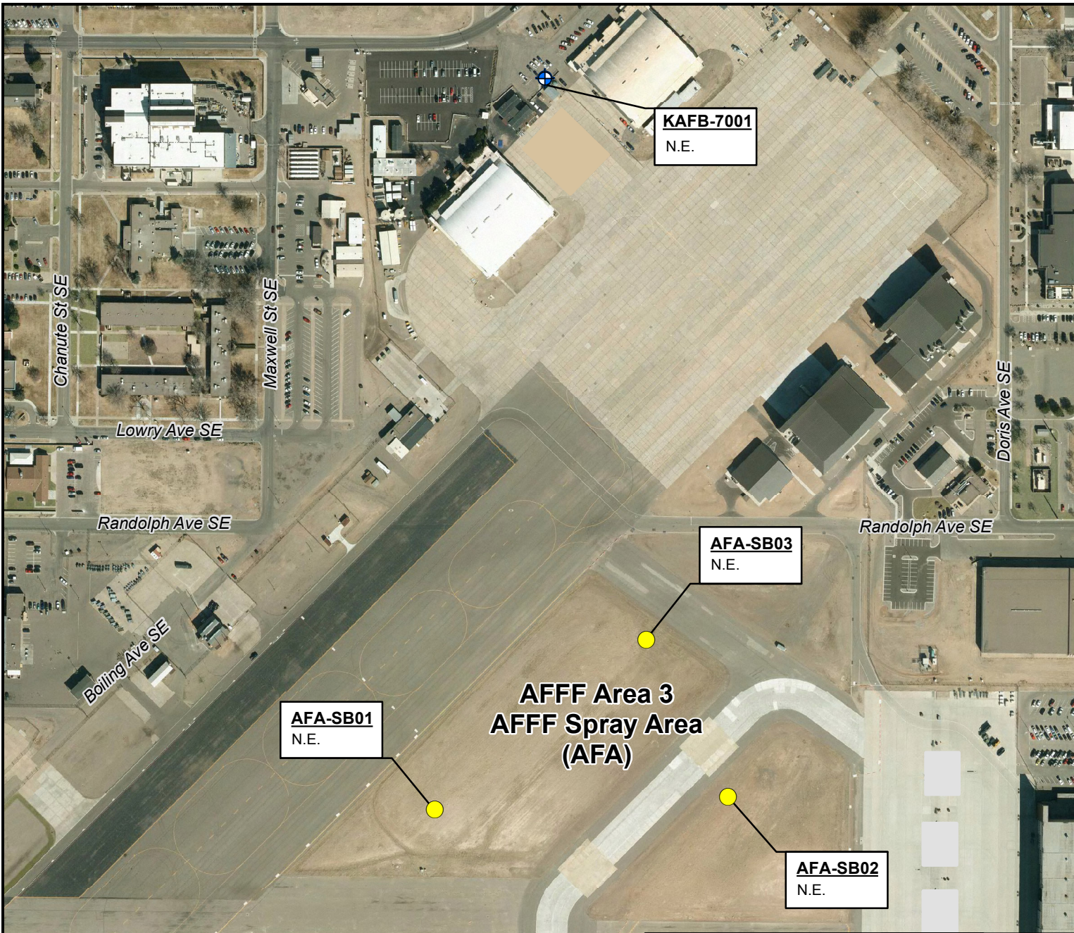
FIGURE 3-4 Sample Locations AFFF Area 3 AFFF Spray Area (AFA) Kirtland Air Force Base Albuquerque, New Mexico
