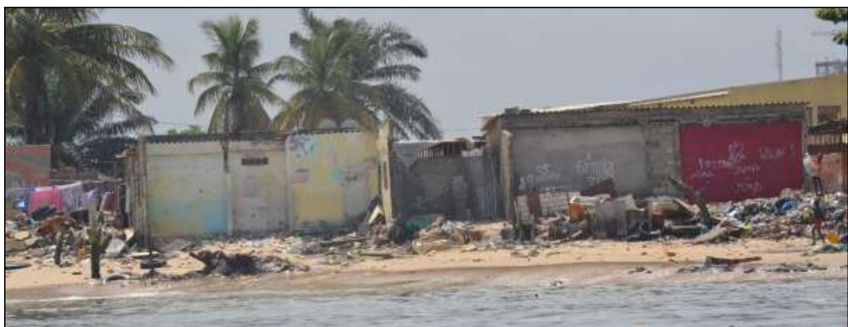
Figure 4.78: Houses damaged by calemas .
