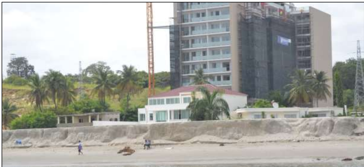
Figure 4.102: Landfill created during the Southwest Marginal works.
