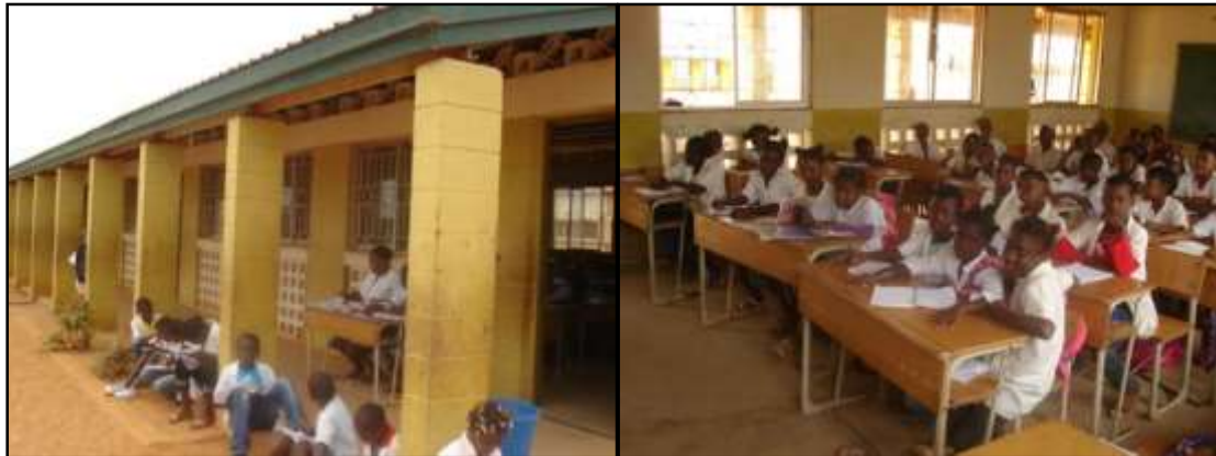
Figure 4.92: Elementary School 1134 (outside). Figure 4.93: Elementary School 1134 (inside).
