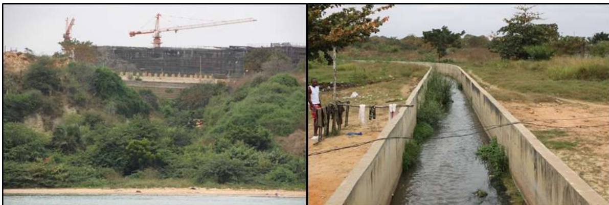
Figure 4.11: Drainage lines existing in the study area. The first image shows a line obstructed by civil engineering works, and the second one, an effluent drainage ditch coming from Talatona.
