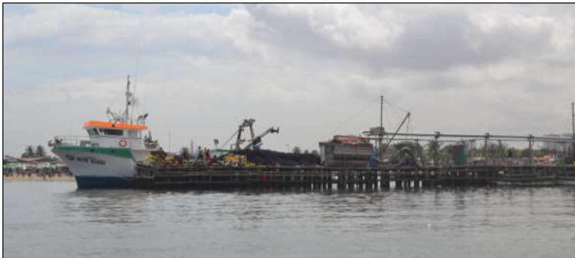
Figure 4.76: Detail of the COAPescas jetty.
