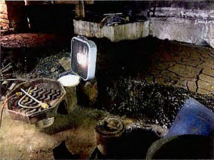
Photo 50: Sludge drying in basement. Note purported F006 listed hazardous waste used as berm material
