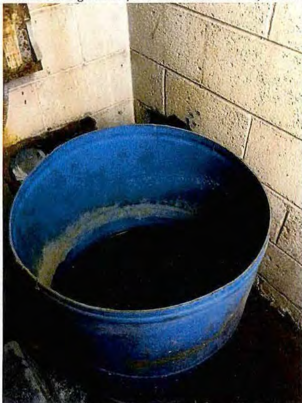
Photo 9: Sewer discharge point
