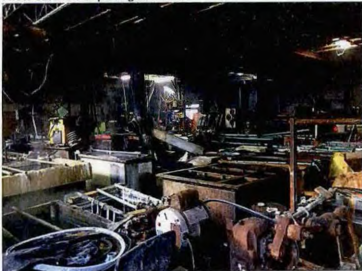
Photo 53: View of plating bath floor
