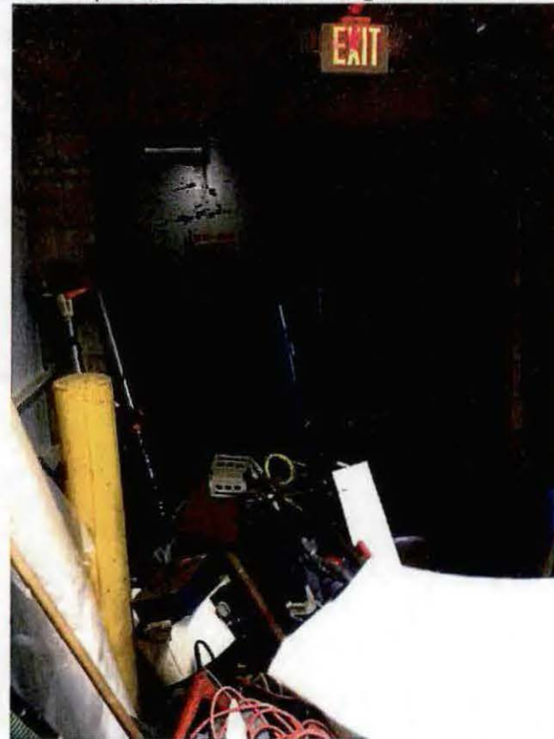
Photo 8: Storage of miscellaneous debris blocking exit
