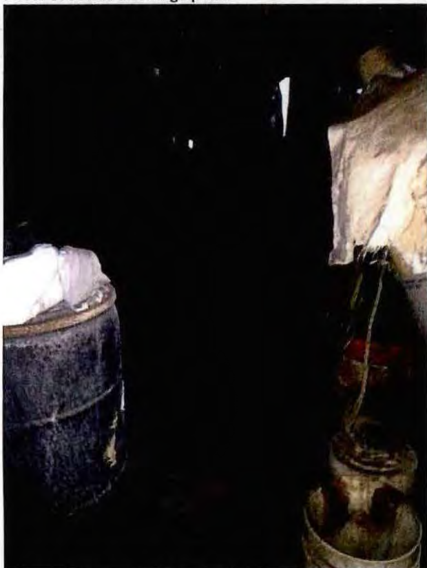
Photo 11: Basement "pit" receiving liquid leakage from plating bath floor above
