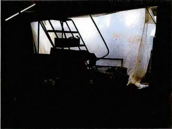
Photo 55: View of missing wall area on top floor of main building
