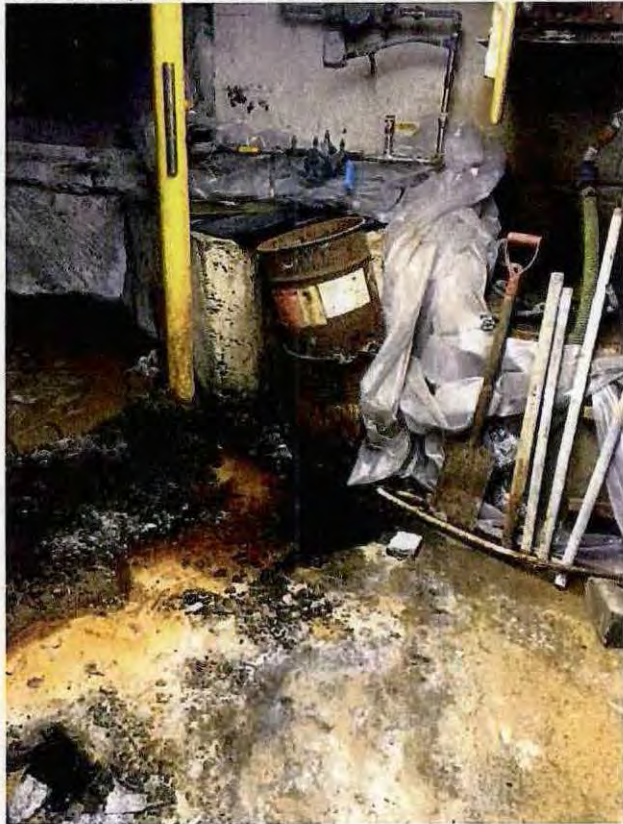
Photo 20: Corroded and leaking containers with "Copper Cyanide" label in basement
