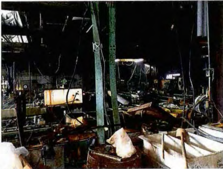
Photo 52: View of plating bath floor
