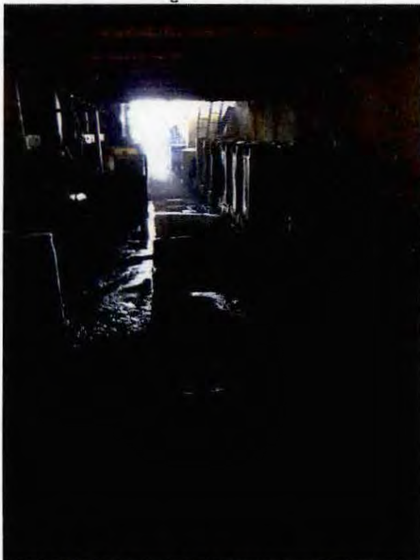
Photo 15: Missing bay door facing north – purported cyanide storage in totes against wall
