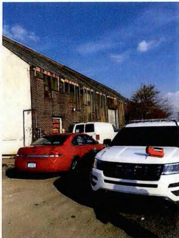
Photo 48: South side of building facing 10 Mile Road
