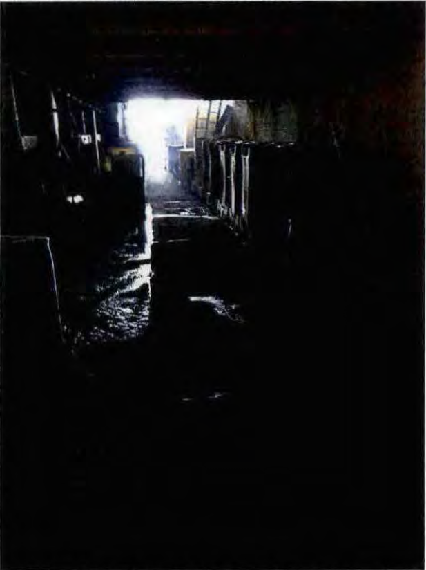
Photo 15: Missing bay door facing north - purported cyanide storage in totes against wall
