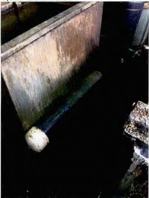
Photo 23: Spilled liquids on plating bath floor
