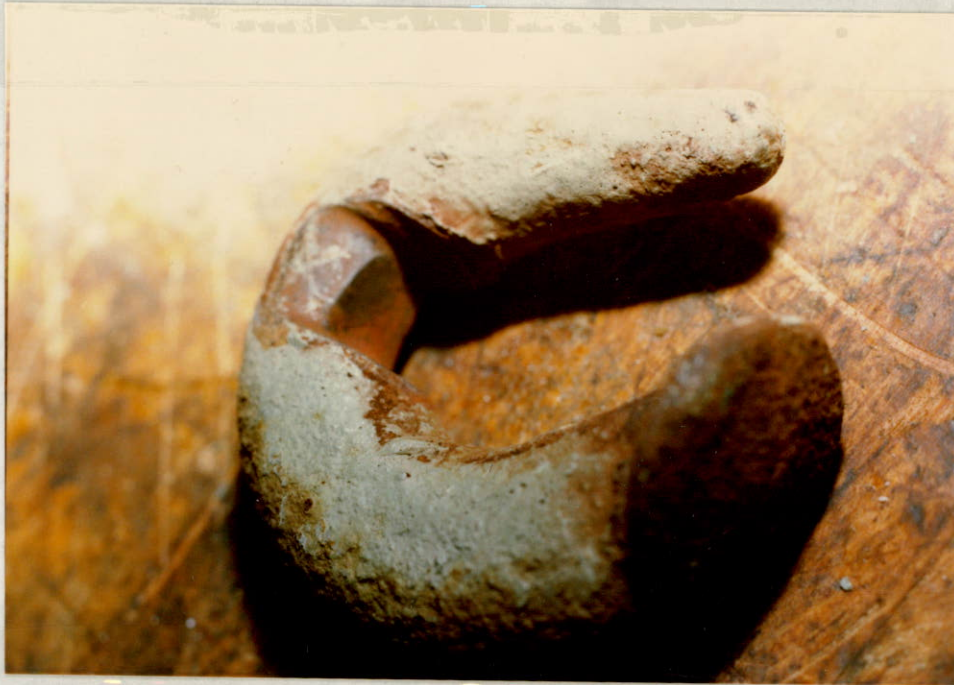
Figure 1. As shown in the Figure above a wear pattern was formed in the bowl-saddle of the J-Hook. This was possibly caused by the insulator string swinging in the wind over a period of time.
