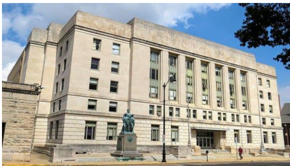
Exterior of the Illinois State Armory Building in downtown Springfield.
