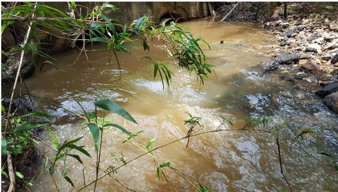
Figure B9 - LDC site for Station 17937
