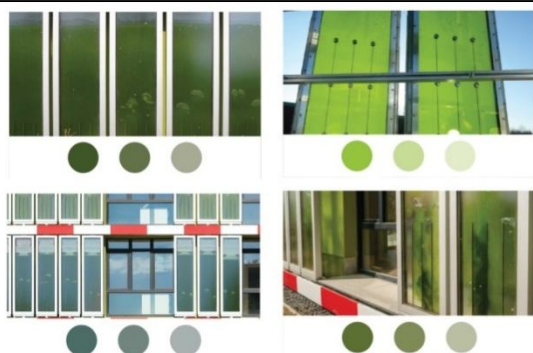
Figure 5. Color Changes for Algal Glass Enclosures (Source: Jo and Han, 2016)
