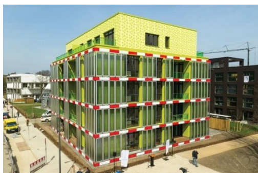
Figure 6. Example for Algal Glass Façade (Source: IBA-Hamburg)
