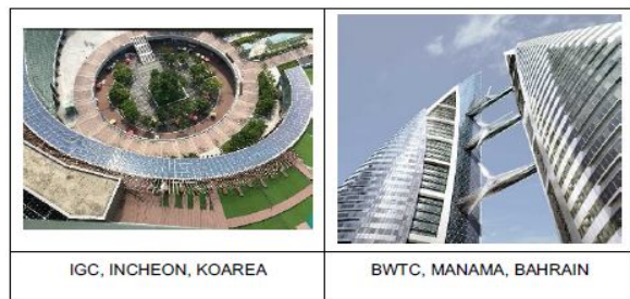
Figure 5. Energy facilities used in buildings
