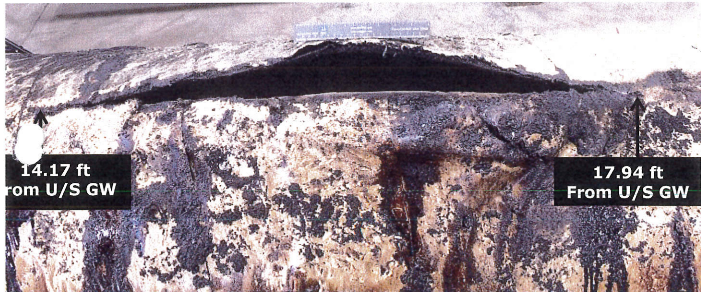
Sections of Pipe Section showing the rupture location following removal of the protective plastic wrappings.
