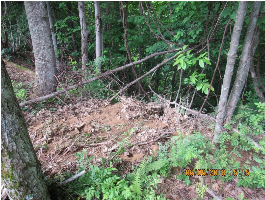
Photo 7: Water leaving the site from control failure at station 6812+58.
