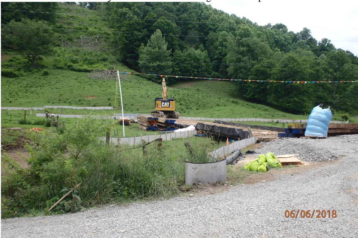
Area adjacent to AR 19 showing BMP installation.
