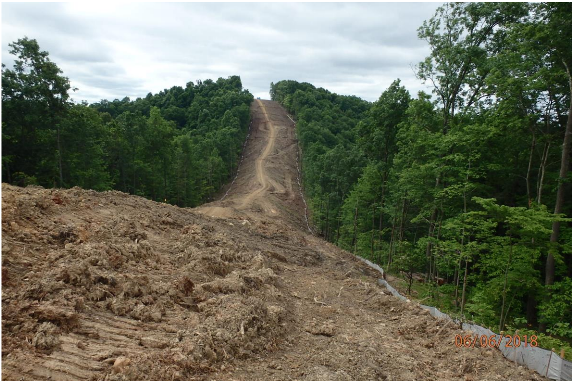
Area adjacent to 498+06 showing controls in place.
