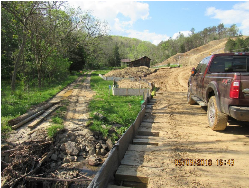
Photo 2: Topsoil delineation, sump, perimeter fencing and vegetative buffer prior to stream.
