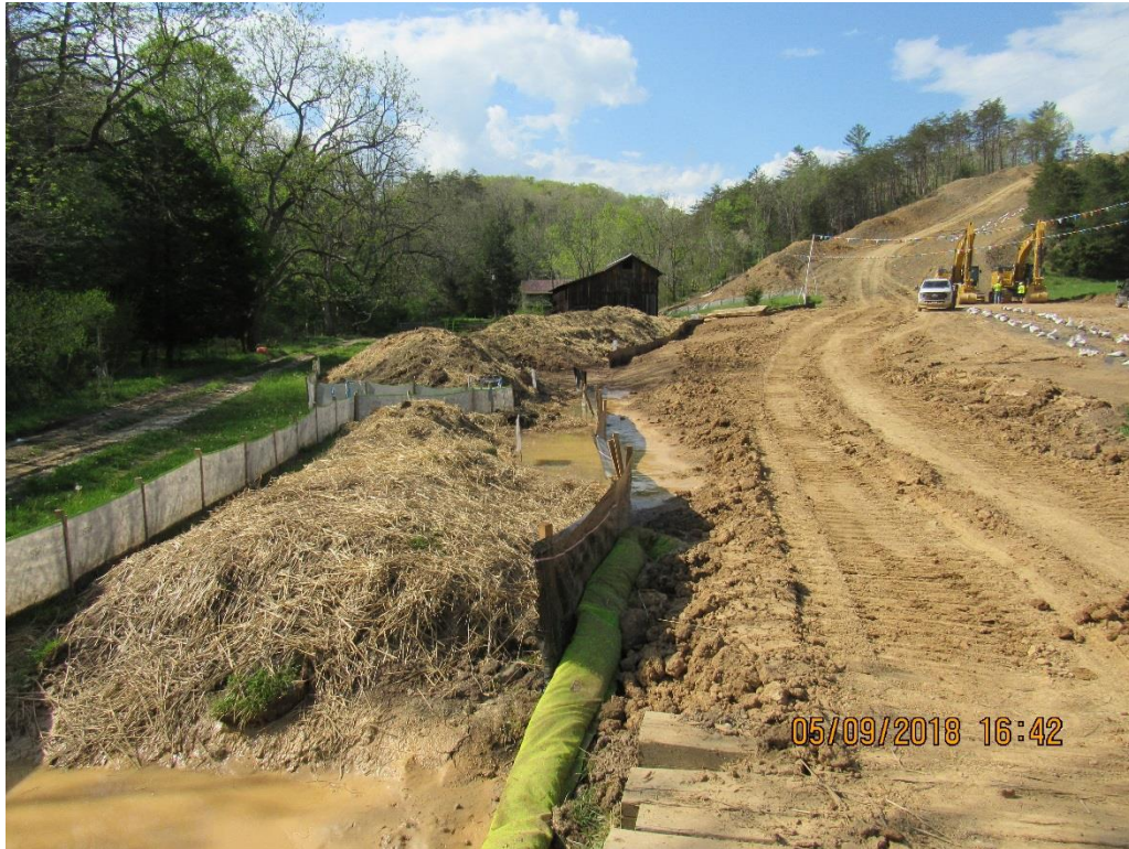
Photo 1: Delineation of topsoil stockpiles from subsoil with black silt fence and path to sump prior to stream.
