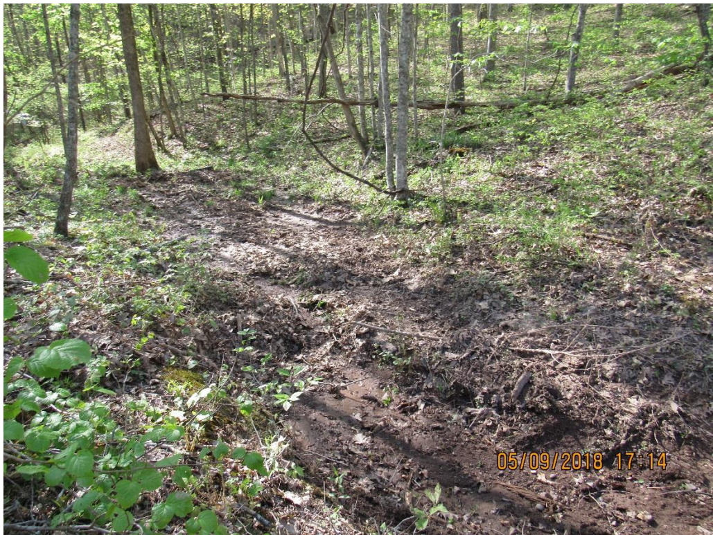
Photo 8: Downstream view of sediment deposits in stream S-IJ65 creating conditions not allowable. (view west)
