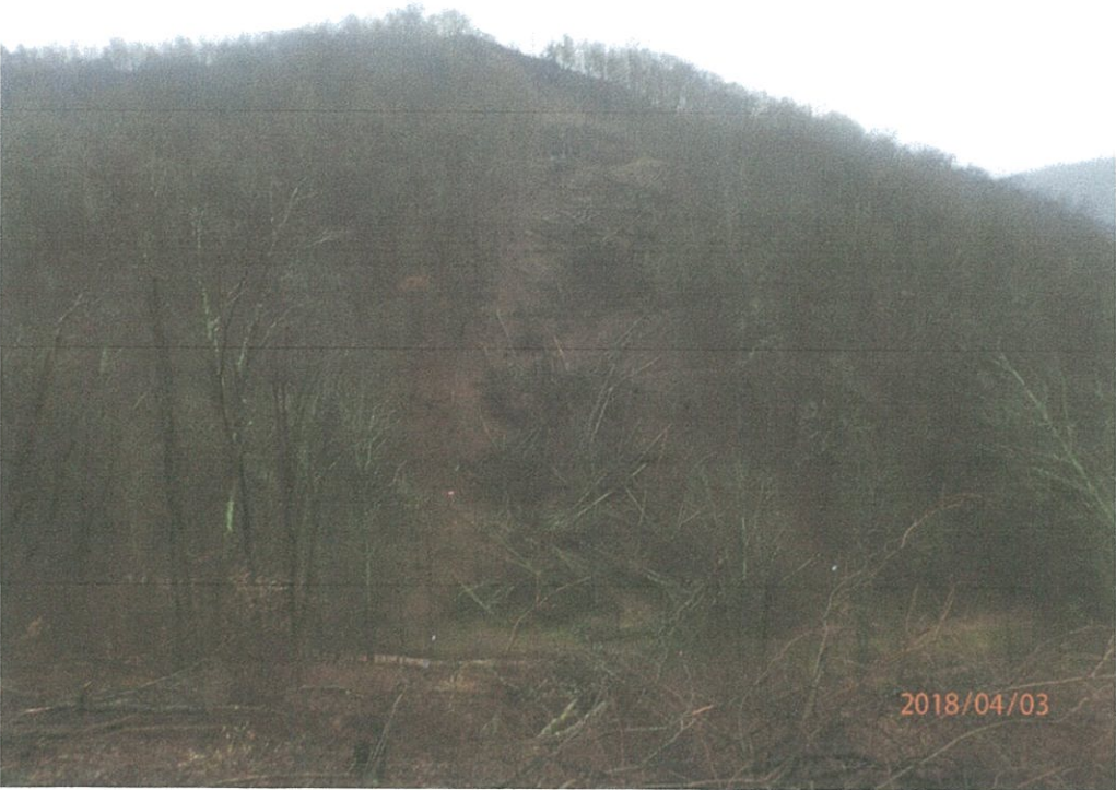
Line clearing off North Fork Road.
