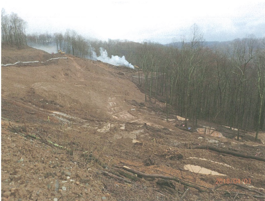
Disturbed area near the reported slip area.
