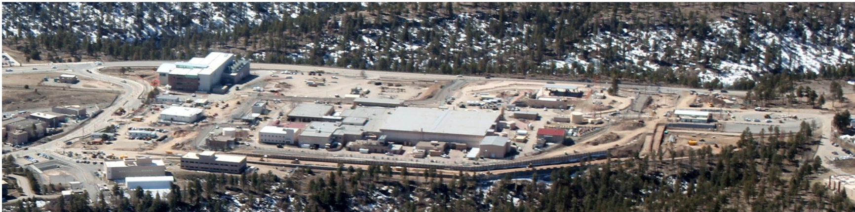
Aerial Photo of TA-55 at LANL, March 2012, showing the absence of any large excavation at the CMRR-NF Site (Los Alamos Study Group)
