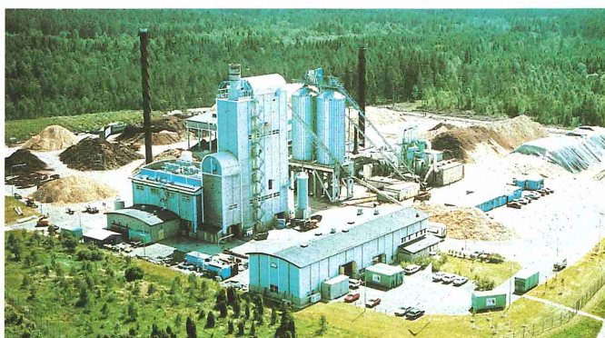
The Värnamo Biomass Plant in Sweden.
