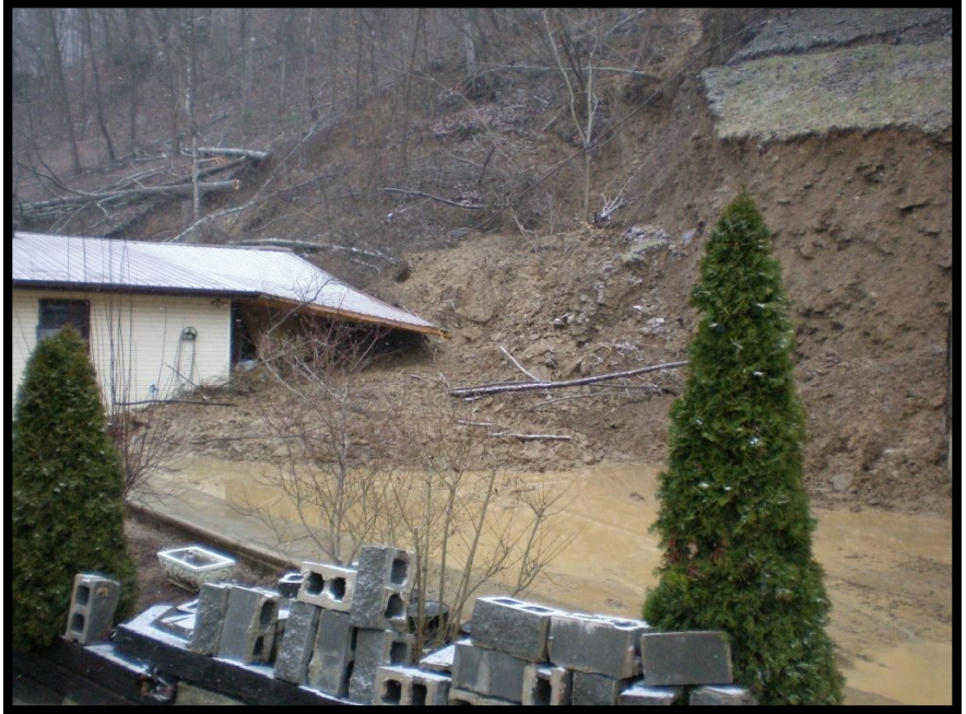
Emergencies such as this one requires AML investigation/ authorization for the repairs to be covered under the new procedures.
