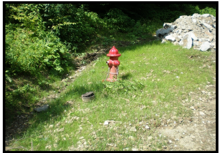
Valve lids, such as this, disappear.
