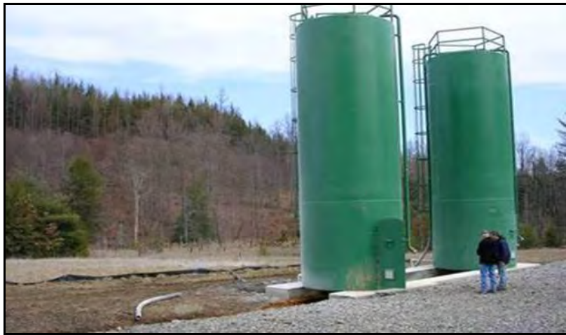
Porcupine Hollow Lime Silos
