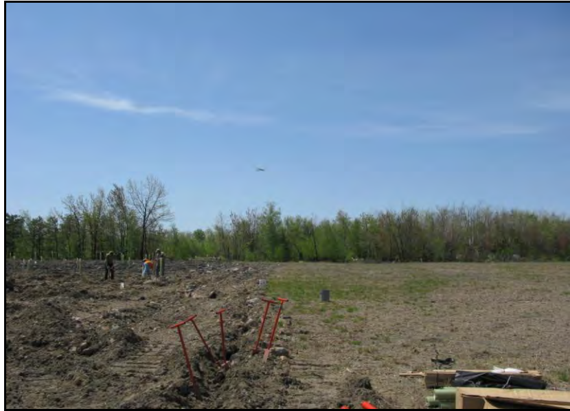
Mountaintop Site showing compacted land on right, and ripped land, suitable for trees on the left
