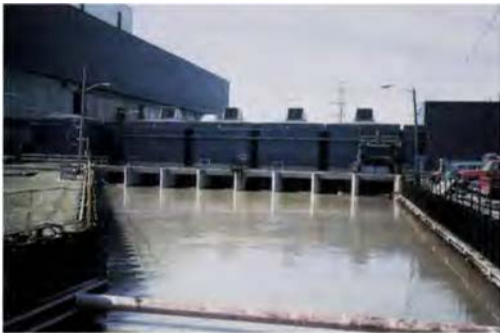
Cooling intake structures
