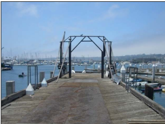
Figure 5-2 Driscoll's Offloading Facility
