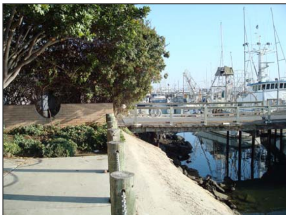
Figure 4-3 Wall interrupting access at Driscoll's Wharf from west
