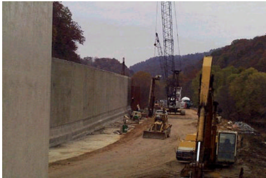
Figure F-9. Floodwall construction to reduce damages
