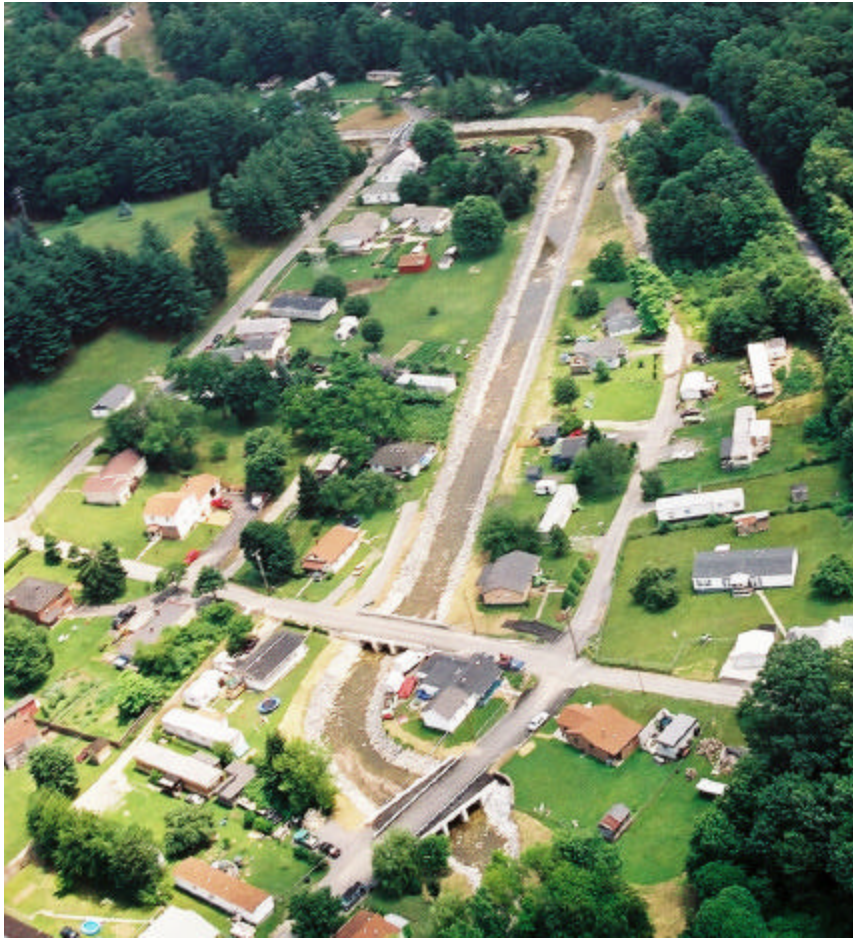
Figure L-7. Little Whitestick Creek channel modification project
