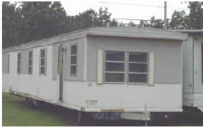
Figure A-1: Unsecured manufactured home
