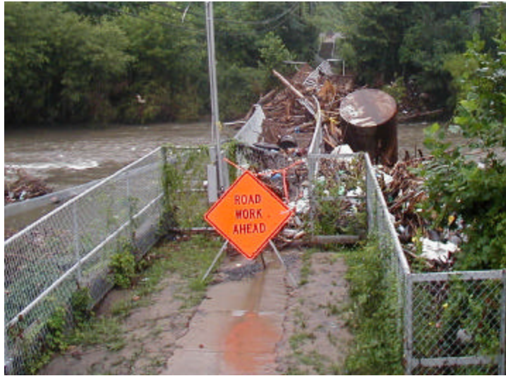
Figure G-2. Abandoned crossing acting as a debris dam after a major flood event
