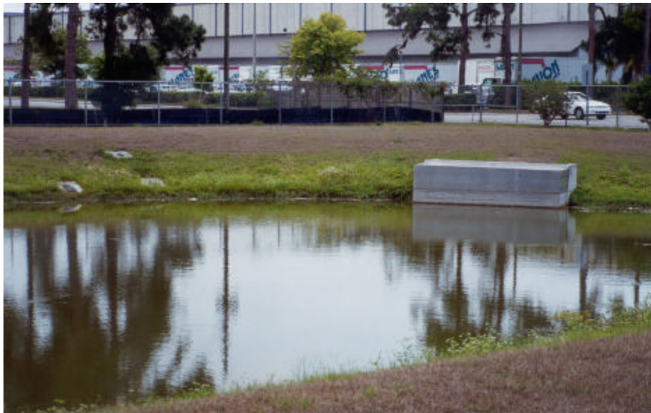
Figure J-7. Stormwater retention facility
