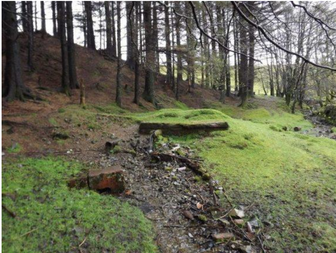
Possible adit structure below B797 road, with 2 outlet pipes, May 2012, (NGR: 287833, 613024)
