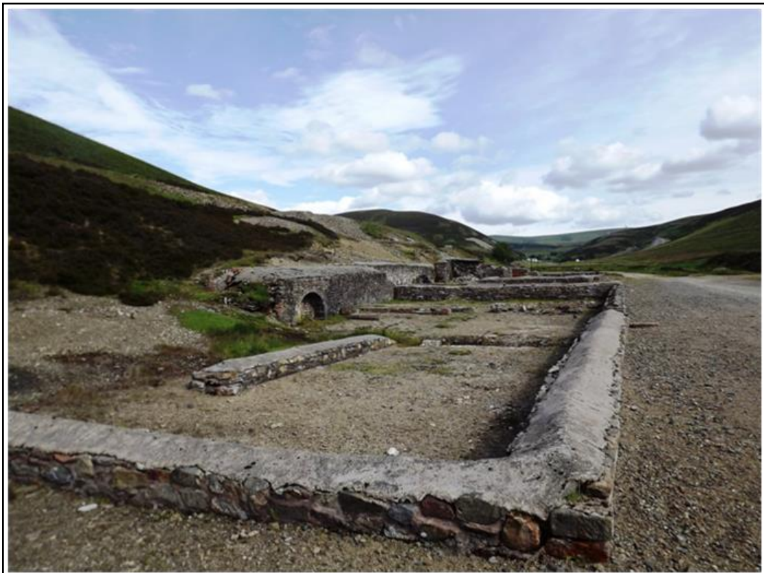
Figure 5.6 – Photo of Queensberry Crushing Mill, looking upstream
