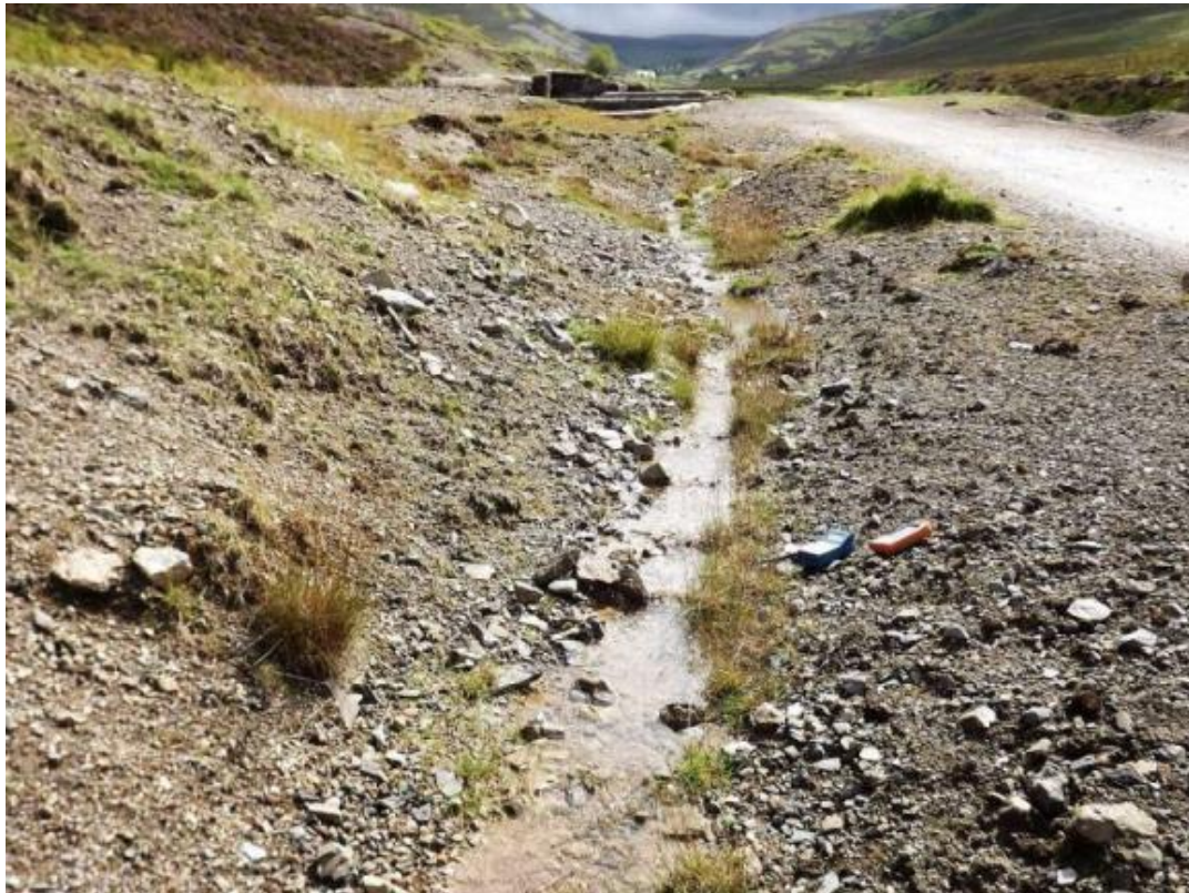
Channel downstream of Queensberry Crushing Mill (in the background), August 2012 (NGR: 285795, 614040)
