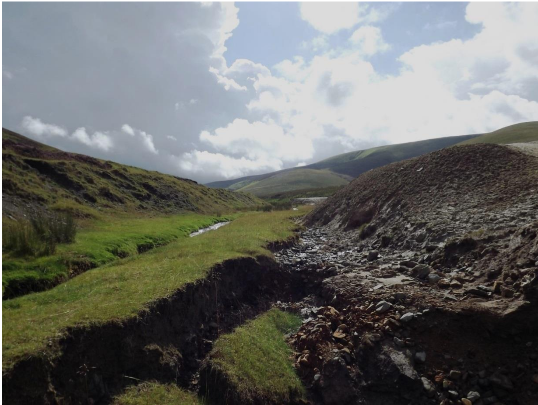
Bank erosion and cutting of the tailings pond area by the Wanlock Water, August 2012.
