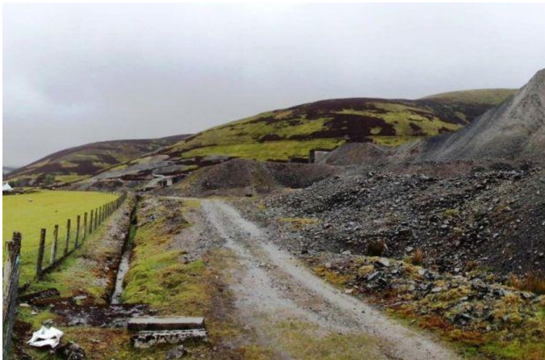
Glencrieff Tip Drain (left) with Glencrieff Mine on the right, May 2012 (NGR: 286416, 613434)
