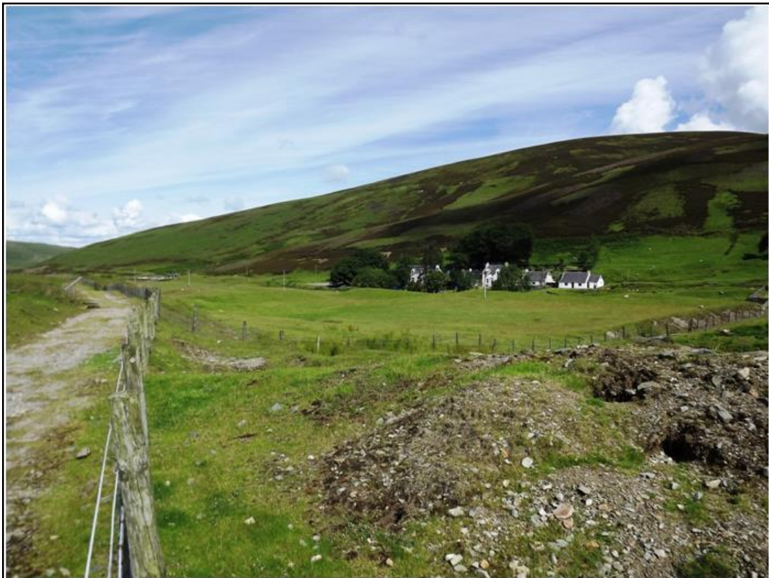
Figure 5.8 – Photo looking towards the area of the grassed covered Glencrieff Settlement Ponds
