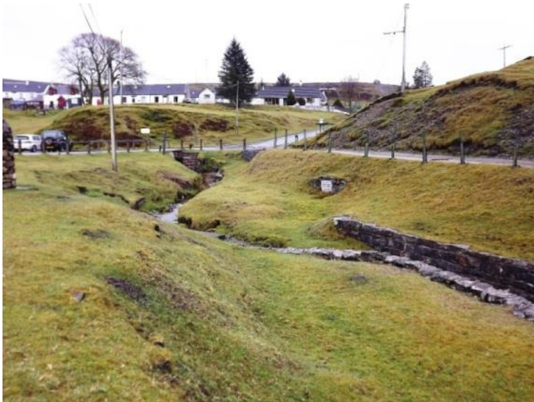
View towards Mennockhass Water Tunnel, May 2012 (NGR: 287300, 612895)
