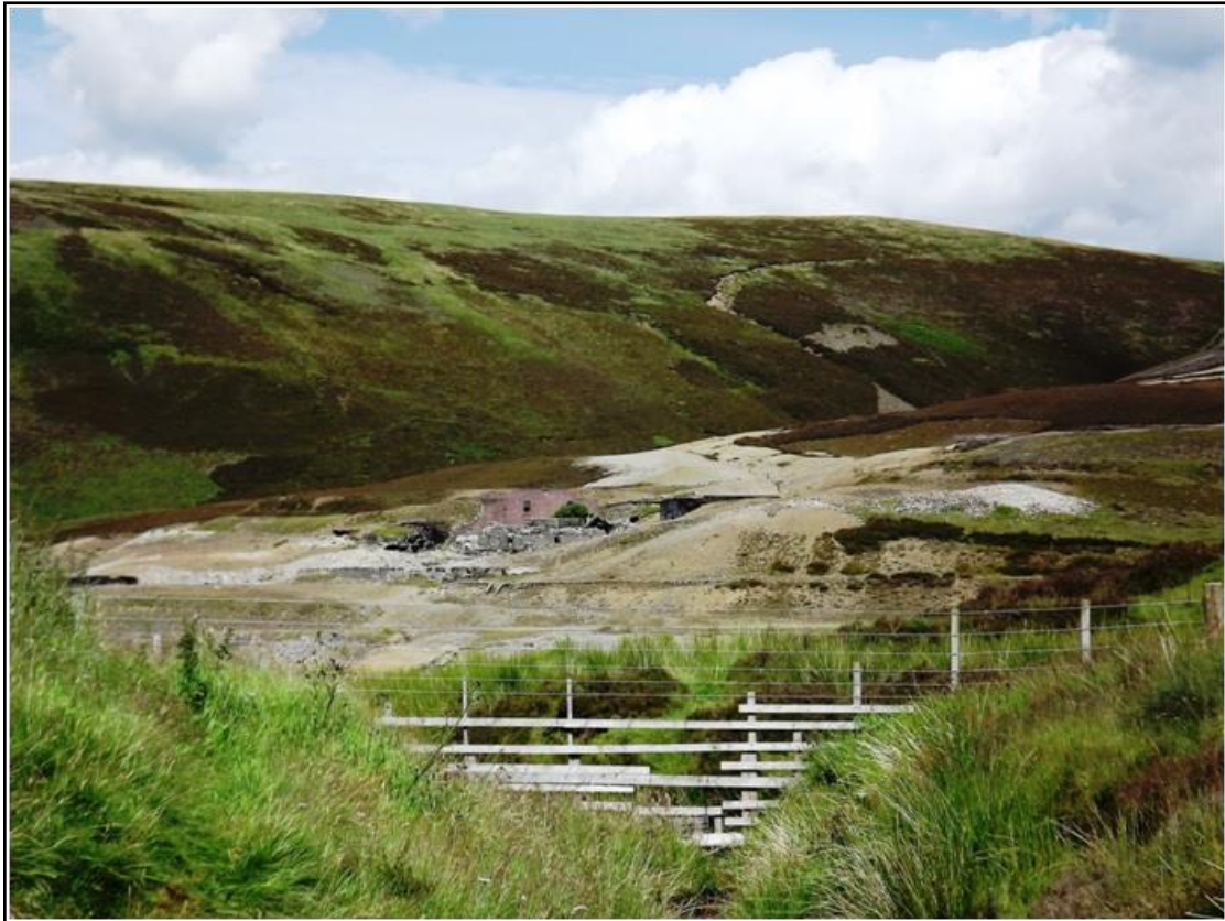
Figure 5.7 – Photo of Queensberry Smelting Mill
