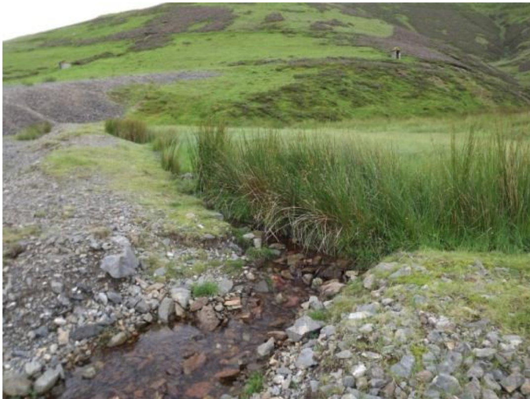
Glenglass Stream outlet from old reservoir above Glencrieff Tip, August 2012 (NGR: 286335, 613335)
