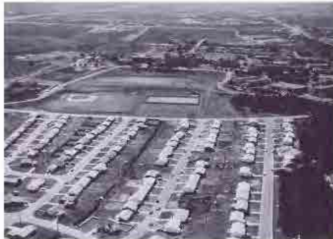
CCIA installed a small drain pipe in the ditch in the late 1960's and levied a fee on the adjacent homeowners to pay for the pipe. As apartment development occurred runoff increased and the drain pipe constantly overflowed flooding homes, streets and property. This is the same scenario occurring in most Central Austin neighborhoods built prior to 1977 where density is being metronized and built with current CDA policies.
