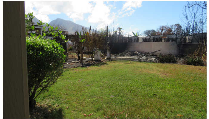
Figure 4.3.4.2.12 Deep yards to the south of (top) 6 and (bottom) 7 Kāua'ula Road separated these surviving structures from destroyed structures to the south. A shed in the southeast corner of 7 Kāua'ula Road was destroyed, yet this fire did not appear to create thermal damage on the main structure.
