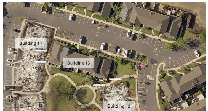
Figure 4.3.3.5.7 Aerial imagery of distances between Building 13 (damaged), Building 12 (destroyed), and Building 14 (destroyed).
