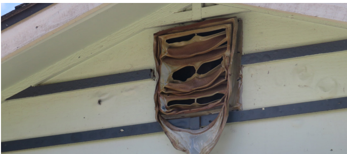
Figure 4.3.4.2.18 Radiant heat damage to the structure and household belongings at 447 Ālīō Street was noted primarily on the north side.
