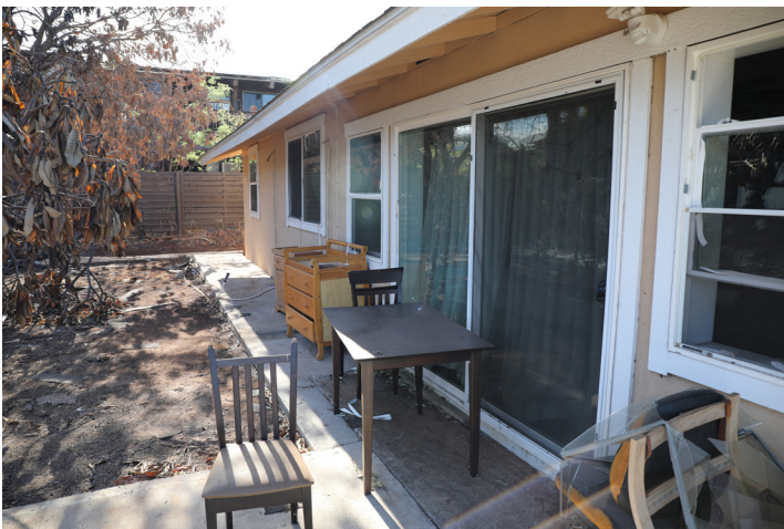
Figure 4.3.5.3.10 The primary structure at 1 Kaniau Road, in close proximity to the destroyed secondary structure and vehicle, had damaged windows, particularly close to the vehicle fire and ember damage to outdoor furnishings that did not extend to the structure.
