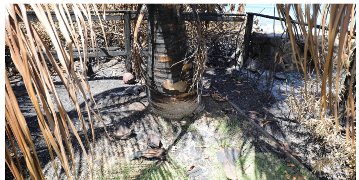
Figure 4.3.4.1.15 Vegetation and fence fire west (makai) of the low stone walls along 4█ and 4█ Front Street. The vegetation fire remained west (makai) of the stone wall other than at the 4█-4█ property line, where a gap is present.
