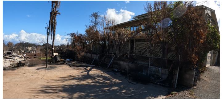
Figure 4.3.5.2.16 12█ 'Ainakea Road (rear view, oriented northeast).
