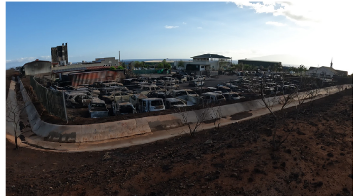
Figure 4.3.5.1.23 Lot of vehicles consumed by fire in the northeast corner of the business park.
