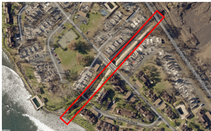
Figure 4.3.4.4.9 Kaua'ula Stream running through Puamana provided a physical separation between the northern section (where structures were destroyed between Hwy-30 and the coast) and the rest of the community (where destroyed structures were limited to the area between Hwy-30 and Pualei Drive).
