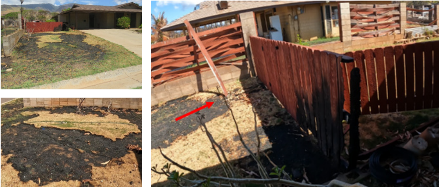
Figure 4.3.4.2.7 Grass fire in the northwest yard of 4█ 'Āli'ō Street appears to have been ignited where charred sections of the fence from the 4█-4█ 'Āli'ō Street property line landed in dry grass, which then backed up to the fence and gate connected to the structure. Sprinklers were distributed throughout the yard, including in the center of this section of undamaged grass.
