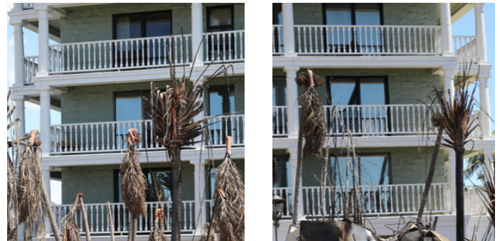
Figure 4.3.4.1.7 Increased window damage on the lower floor windows on the west-makai (right) compared to the east-mauka (left). Cracking is noted on the second and fourth floor windows with screens partially dropped on the third and fourth floors for the rooms on the west (makai).
