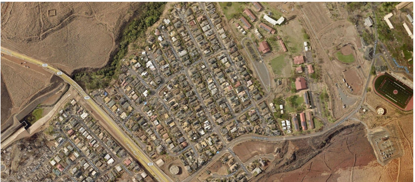
Figure 4.3.3.2.1 Post-fire aerial imagery Kelaweia Mauka III subdivision, east (mauka) of Lahaina Bypass.
