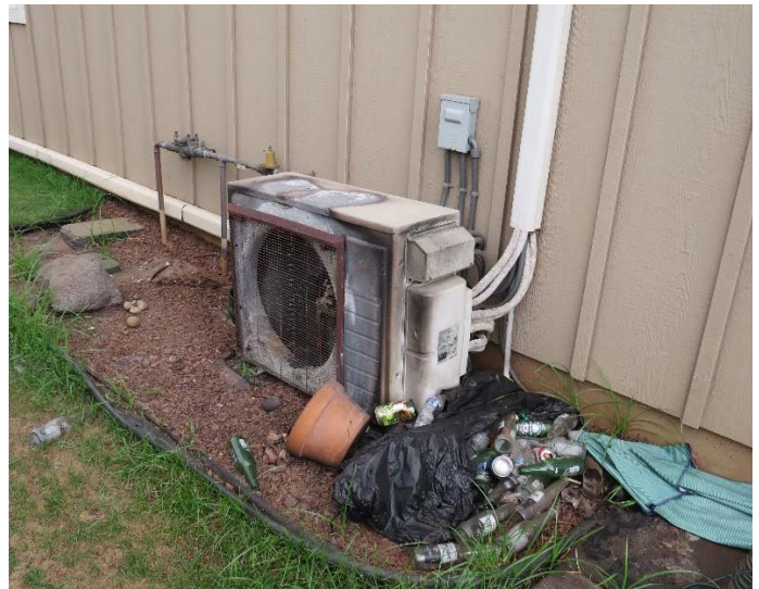
Figure 4.3.3.3.4 Isolated fire damage to 311 Komo Mai Street. Spot fire (ember ignition) caused localized damage, but did not spread to the structure, likely due to defensive actions.
