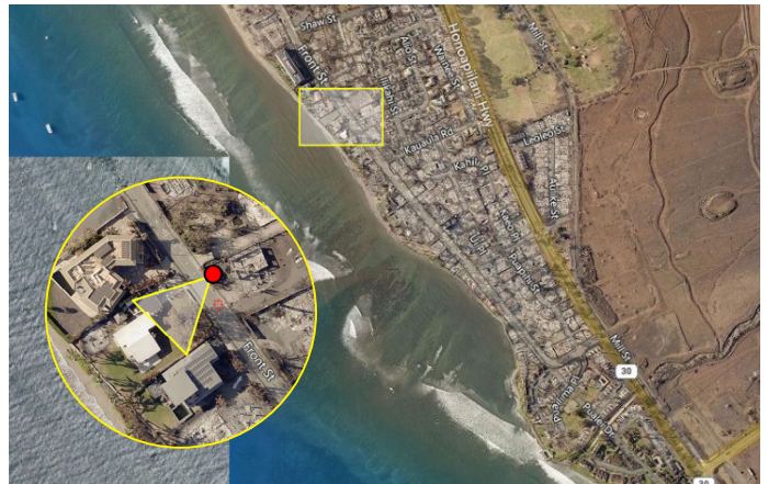
Figure 4.3.4.1.12 Debris in the open garage of 4 Front Street. Inset: Viewpoint showing the area depicted in the photograph above.
