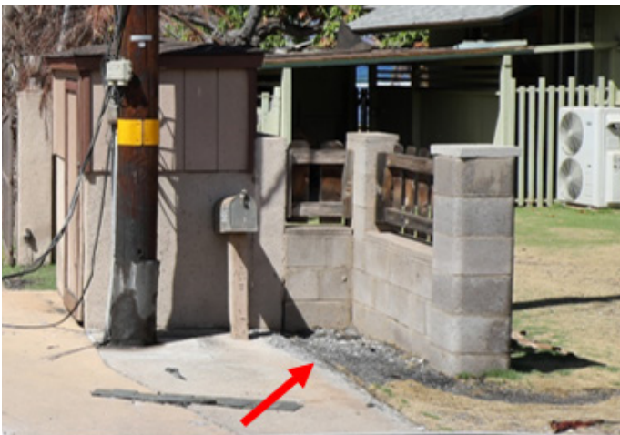
Figure 4.3.4.3.4 Tall, lush vegetation was planted along block walls on either side of the driveway to 3█ Front Street, which may have provided protection to the 3█ and 3█ Front Street lots. The block wall south of 3█ Front Street also influenced the ember movement. Note pile up in corner of wall (bottom left) and wind driven burn scar in grass around the wall toward the front of the structure showing the likely path of ground based embers deflected towards the north and away from the open garage (bottom right).
