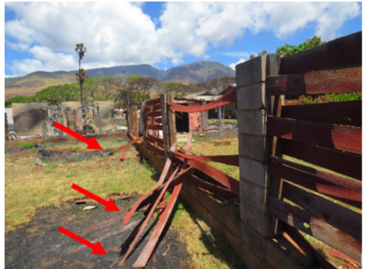
Figure 4.3.4.2.6 Grass fire to the south of 4 th 'Ālī'ō Street appears to have ignited in multiple locations where charred sections of the fence from the 4 th -4 th 'Ālī'ō Street property line landed in dry grass. While it propagated near the wooden structure on the southside of 4 th 'Ālī'ō Street, it did not transition to the structure.
