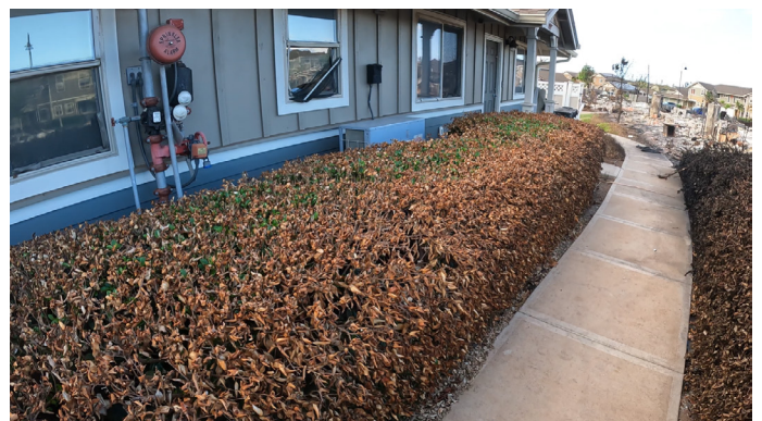
Figure 4.3.3.5.8 Ground-based photograph of space between Building 13 (shown on the left of the image) and Building 14 (shown on the right), showing damaged windows and heat damaged/dried (but not ignited) vegetation.
