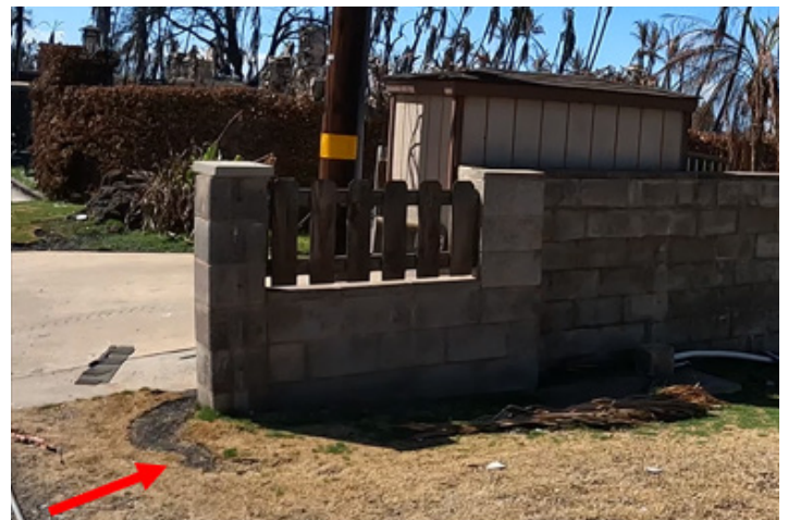
Figure 4.3.4.3.4 Tall, lush vegetation was planted along block walls on either side of the driveway to 3█ Front Street, which may have provided protection to the 3█ and 3█ Front Street lots. The block wall south of 3█ Front Street also influenced the ember movement. Note pile up in corner of wall (bottom left) and wind driven burn scar in grass around the wall toward the front of the structure showing the likely path of ground based embers deflected towards the north and away from the open garage (bottom right).
