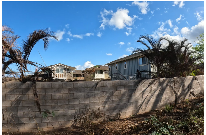
Figure 4.3.3.5.6 Destroyed single family home from the rear on the other side of the concrete wall.
