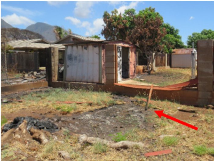
Figure 4.3.4.2.6 Grass fire to the south of 4 th 'Ālī'ō Street appears to have ignited in multiple locations where charred sections of the fence from the 4 th -4 th 'Ālī'ō Street property line landed in dry grass. While it propagated near the wooden structure on the southside of 4 th 'Ālī'ō Street, it did not transition to the structure.
