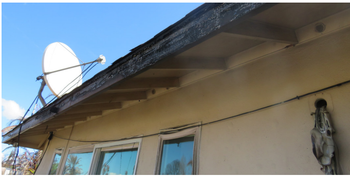
Figure 4.3.4.2.15 West (makai) side of 6█ Kaua'ula Road withstood extensive damage to windows, including three (3) casement style windows where frames were severely warped and both panes of glass failed and dropped out of the frame. The interior screen remained in place for all three (3) windows, and appears to have blocked some materials from entering the structure.
