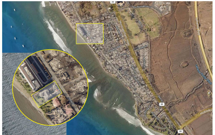
Figure 4.3.4.1.10 Ember and/or radiant heat ignited and destroyed the 475 Front Street garbage can/disposal area, which subsequently damaged a light post and the wood railing/fence on the northwest corner of 4 Front Street. Inset: Viewpoint showing the area depicted in the photograph above.
