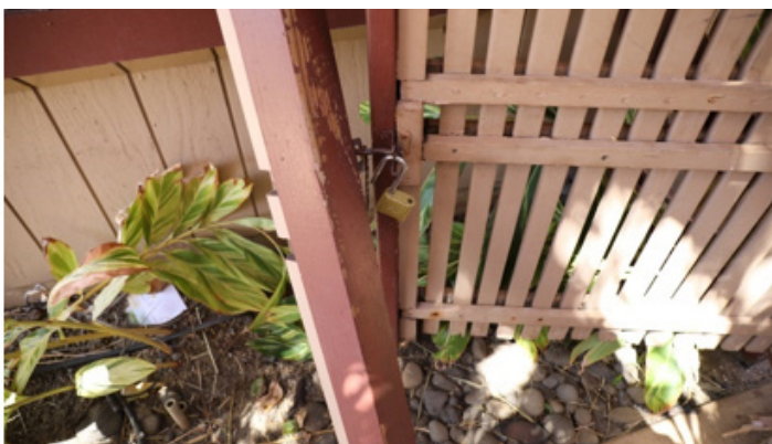
Figure 4.3.4.3.8 Gate and post moved away from burning fence pickets that interrupted the continuous wooden fuel from the 3█-3█ property line to the east (mauka) wall of 3█ Front Street. The charred end of the post remaining in the ground is indicated by the red arrow in the bottom right image.
