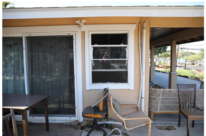
Figure 4.3.5.3.10 The primary structure at 1 Kaniau Road, in close proximity to the destroyed secondary structure and vehicle, had damaged windows, particularly close to the vehicle fire and ember damage to outdoor furnishings that did not extend to the structure.
