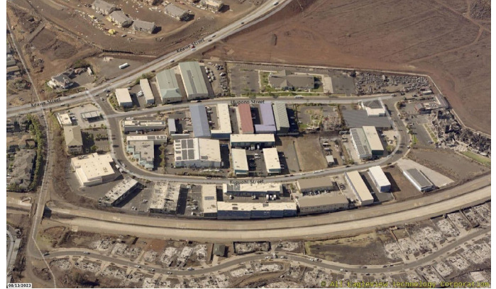
Figure 4.3.5.1.1 Post-fire aerial imagery of Lahaina Business Park.
