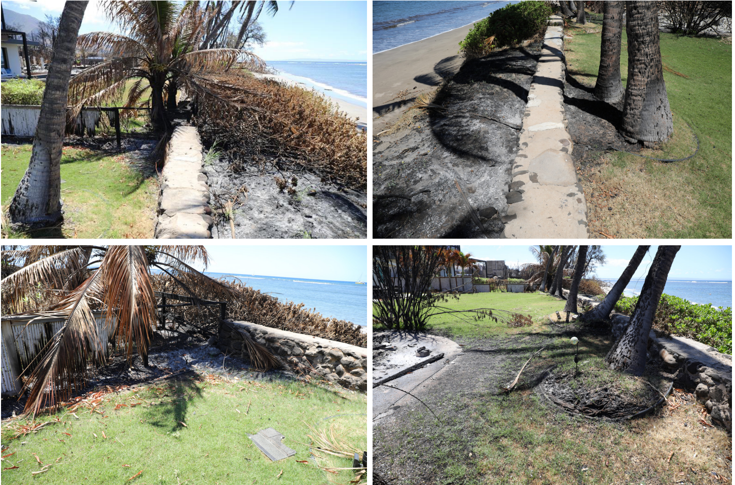
Figure 4.3.4.1.16 Vegetation fire west (makai) of the property line for 4█ Front Street appears to cross into the backyard at the 4█-4█ Front Street property fence line and near large trees proximate to the wall. Note destroyed accessory structure to the left of the bottom, right image.
