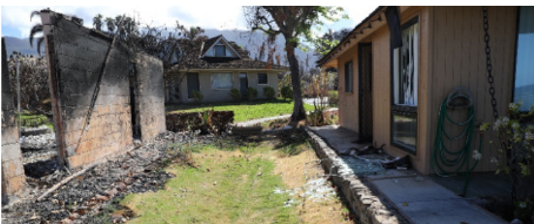
Figure 4.3.4.4.8 Damage to the north end of 4 Pualoke Place immediately adjacent to the destroyed structure at 3 Pualoke Place. A tree to the east (mauka) of the structure sustained deep charring, likely from embers gathering in cracks, fissures, or scars in the tree bark (top left). Window damage on the north structure wall (top right) ranges from single pane cracking to vinyl frame warping (middle left) to complete pane fallout (middle center). Plastic vent cover and gutters melted and fell. Paint bubbled and peeled across most of the surface. No apparent indication of charring or damage to wood shake roofing materials or wood wall substrate (top right and middle right). Grass remained green between the destroyed and damaged structure. Garden hose noted at the corner of the structure (bottom left). Inset: Viewpoint showing area shown in the photographs above.
