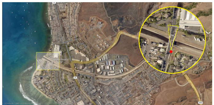
Figure 3.8.2.2 Northbound Front Street traffic over Kahoma Stream on August 8, 2023, at 17:05. Inset: Viewpoint of northbound Front Street traffic over Kahoma Stream on August 8, 2023, at 17:05.
