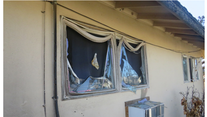
Figure 4.3.4.2.15 West (makai) side of 6█ Kaua'ula Road withstood extensive damage to windows, including three (3) casement style windows where frames were severely warped and both panes of glass failed and dropped out of the frame. The interior screen remained in place for all three (3) windows, and appears to have blocked some materials from entering the structure.
