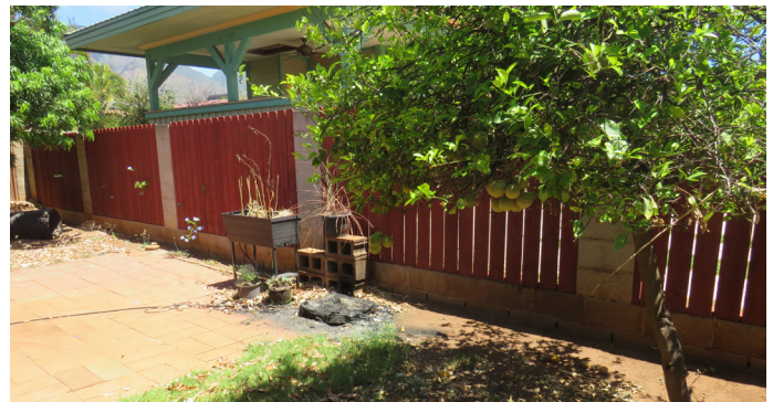
Figure 4.3.4.2.7 Grass fire in the northwest yard of 4█ 'Āli'ō Street appears to have been ignited where charred sections of the fence from the 4█-4█ 'Āli'ō Street property line landed in dry grass, which then backed up to the fence and gate connected to the structure. Sprinklers were distributed throughout the yard, including in the center of this section of undamaged grass.
