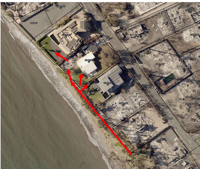
Figure 4.3.4.1.14 Overhead view of 4█-4█ Front Street showing potential path of fire progression along a low stone wall west (makai) of the property lines and then east (mauka) along 4█-4█ property line wood fence, into an accessory structure and a chair by on the patio of 4█ Front Street (see Figures 4.3.4.1.15, 4.3.4.1.16, 4.3.4.1.17, 4.3.4.1.18).
