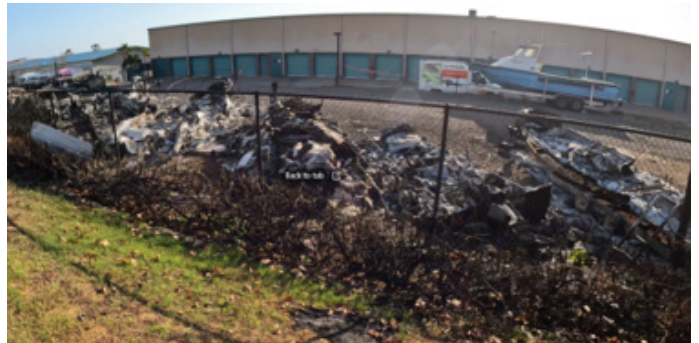
Figure 4.3.5.1.11 Vehicles consumed by fire west (makai) of the church (8█ Ulupono Street).
