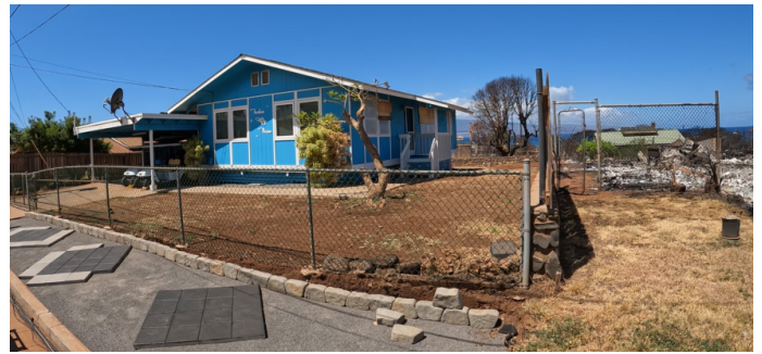
Figure 4.3.5.2.10 12█ Nahale Street on the left and 12█ Nahale Street (destroyed) on the right.
