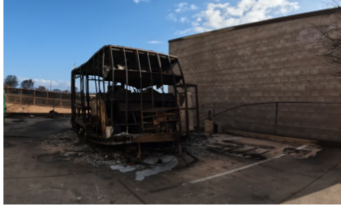
Figure 4.3.5.1.8 Trailer and building materials ignited by embers (1█ Kupuohi Street).
