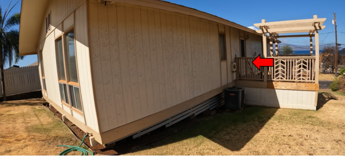
Figure 4.3.5.2.12 Northeast corner of 12█ 'Ainakea Road with blistering paint from radiant heat exposure (indicated by red arrow).
