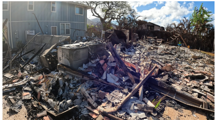
Figure 4.3.3.5.4 Destroyed single family home at 2█ Kahoma Village Loop from the front (north).
