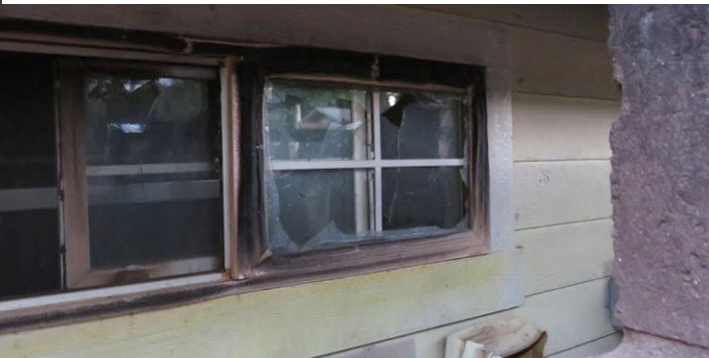
Figure 4.3.3.6.4 Destroyed accessory structure at 4 Ala Moana Street (top left). The burning structure caused damage to 4 Ala Moana Street (top right and bottom left) and 5 Ala Moana Street (bottom right).
