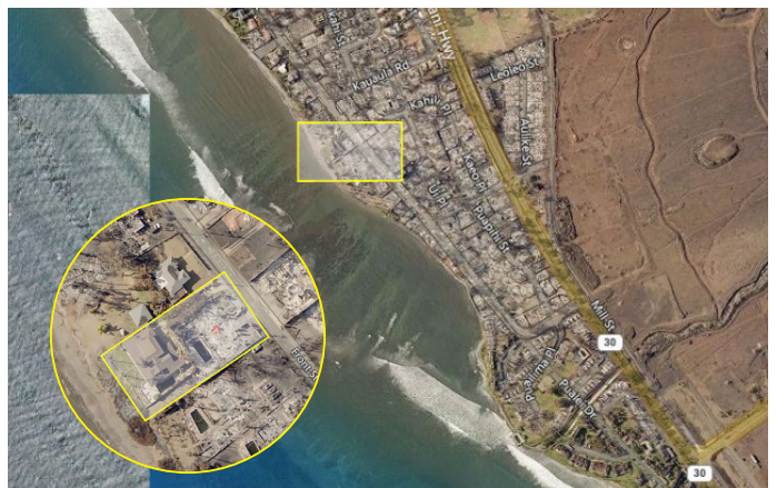
Figure 4.3.4.3.5 The east (mauka) facing exterior wall of 3█ Front Street did not have any indication of radiant heat damage and there were relatively limited signs of embers along the ground. Tall, lush vegetation plated along a block half-wall between 3█ and 3█ Front Street was still standing, including some plants that remained green at the time of the post-fire analysis. Inset: Viewpoint showing the area depicted in the photographs above.
