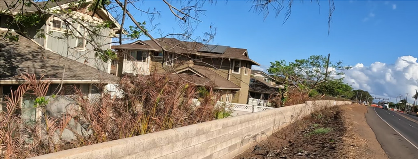
Figure 4.3.3.5.3 Concrete barrier wall along Hwy-30.
