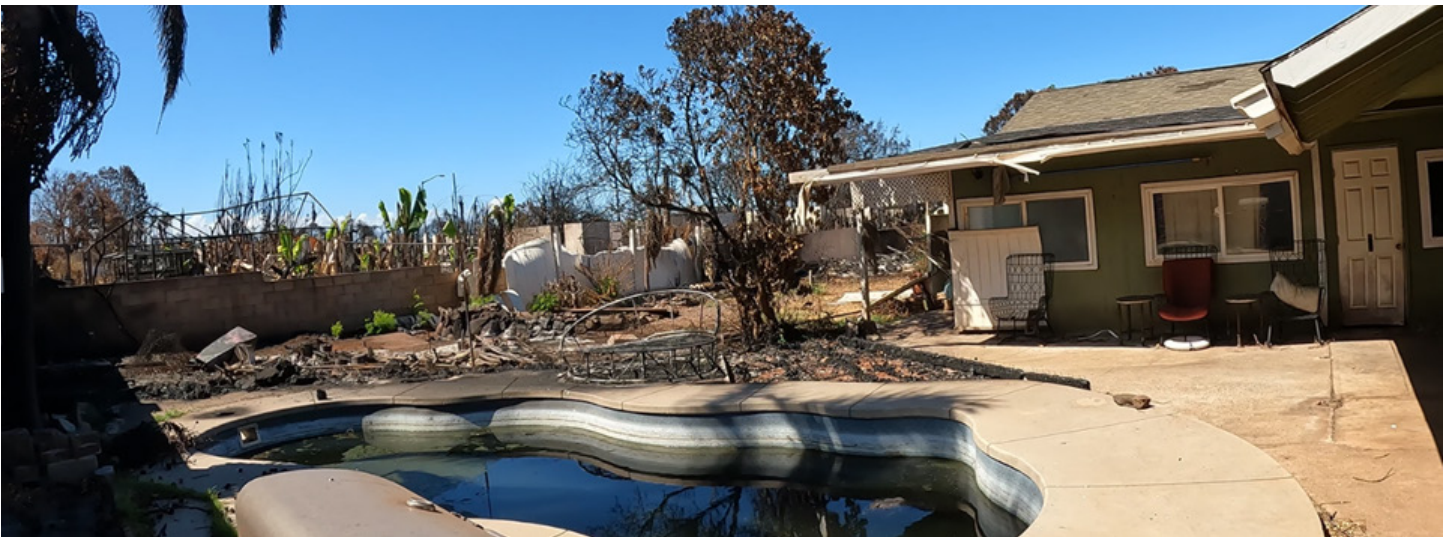
Figure 4.3.4.2.13 Exterior fire in the south yard of 7 Kāua'ula Road destroyed outdoor furnishings and structures up to the corner of the main residential structure. However, these fires did not spread to the south of the residence and appeared to result only in damage to the plastic gutter in the southwest corner.
