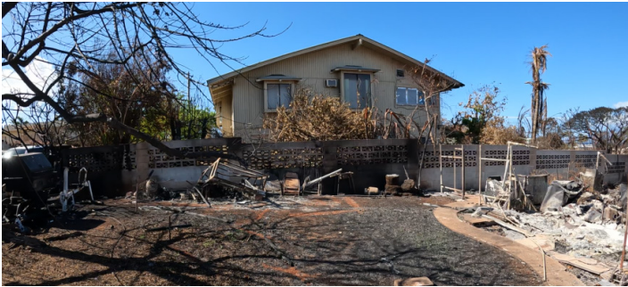
Figure 4.3.5.2.15 12█ 'Ainakea Road (side view, oriented north).
