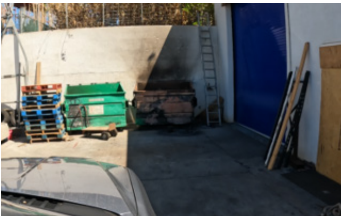
Figure 4.3.5.1.15 Dumpster fire to the west (makai) of 2 █ Kupuohi Street.
