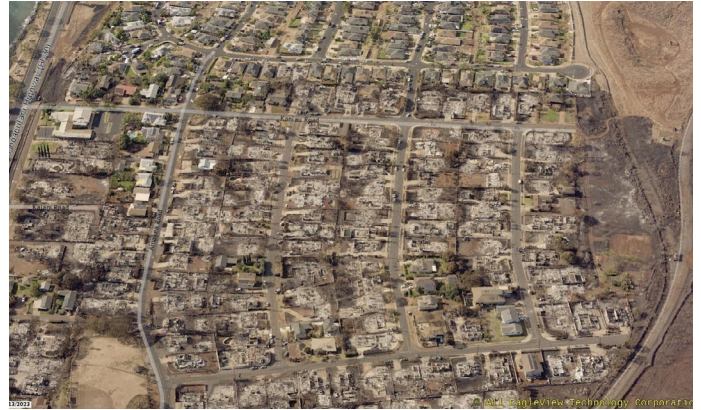
Figure 4.3.5.3.1 Aerial imagery of the North Zone, between Kaniau Road and 'Aipuni Street, which is the most northern area of Lahaina affected by the August 2023 Maui fires.
