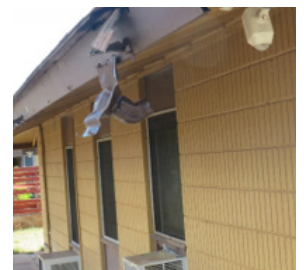
Figure 4.3.4.2.5 Eave and roof damage to the structure at 4█ ‘Ālī’ō Street.
