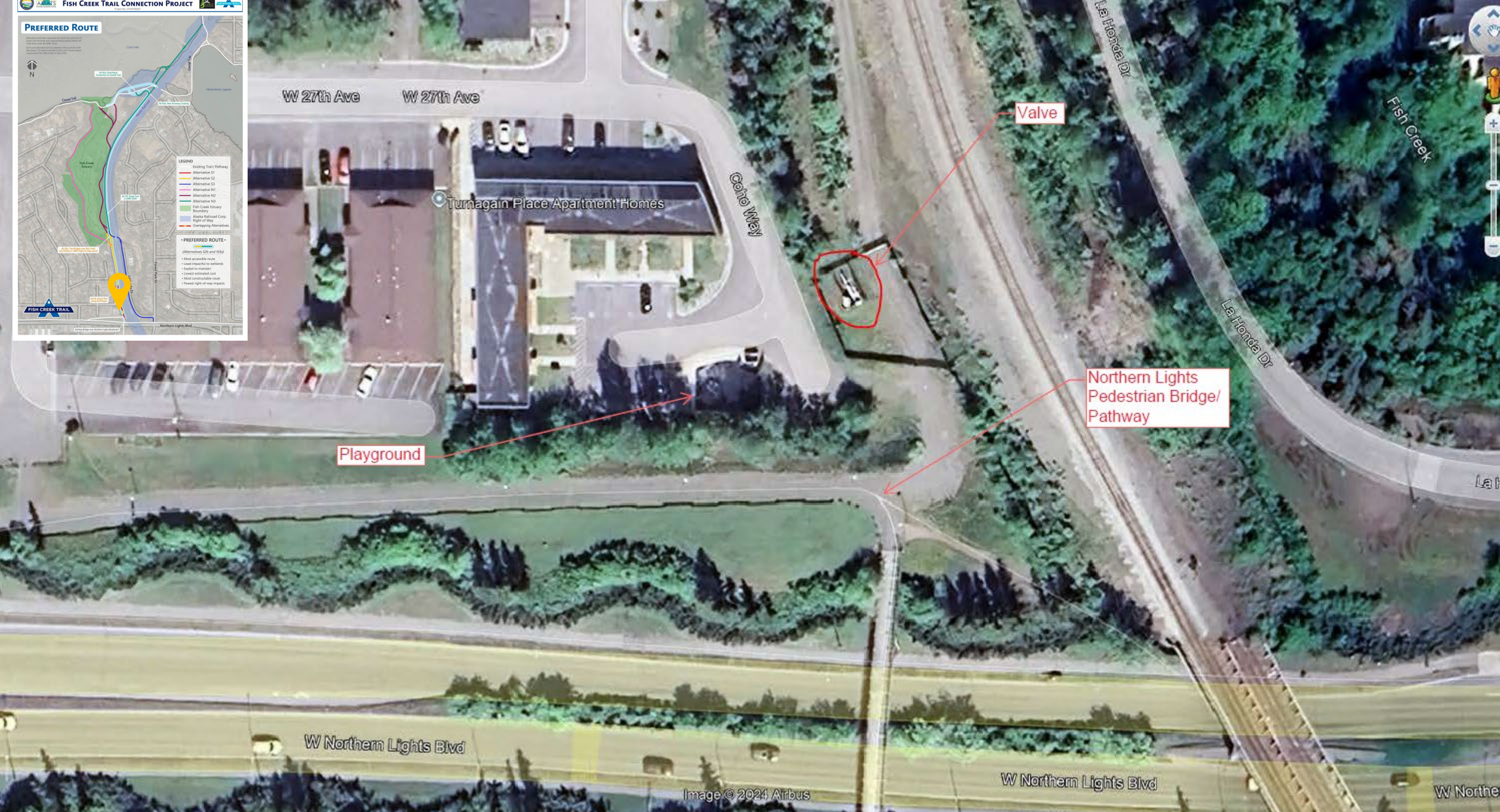
Bird's eye view of the valve adjacent to both the railroad tracks and a ROW used to access a residential area.
