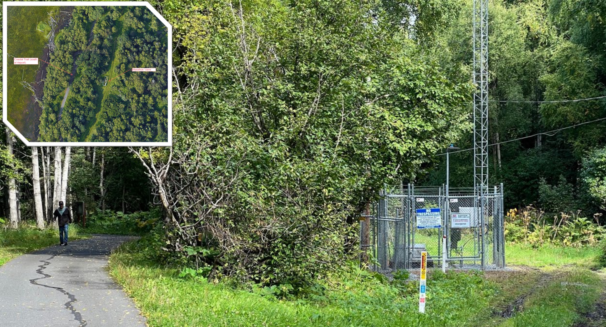
This is an existing valve adjacent to the coastal trail , and an example of the utility and a similar trail coexisting.
