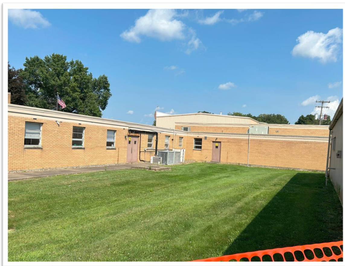
Figure 5: Photo of the alcove and A/C unit by which Crooks gained access to the AGR roof 246
