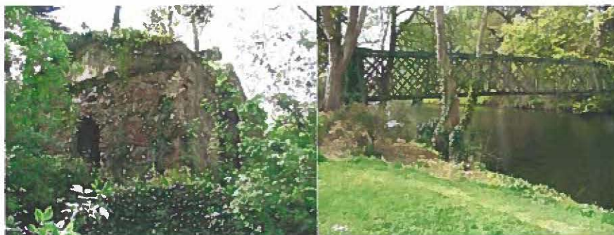
L-R: Bath house, and steelwork bridge (Source: NIAH)
