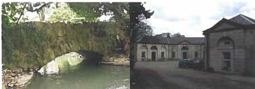
L-R: Stone bridge and stable building (Source: NIAH)
