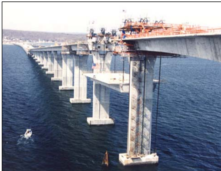
Figure 3.11. Heavy-Lift Construction (Jamestown-Verrazanno Bridge)
