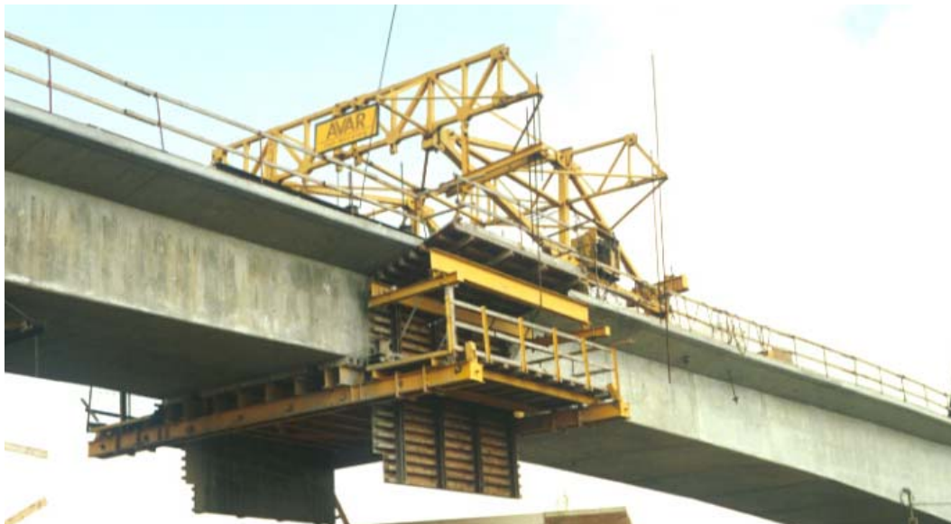
Figure 3.17. Casting of Closure Segment (Kramer-Rosecrans Bridge)
