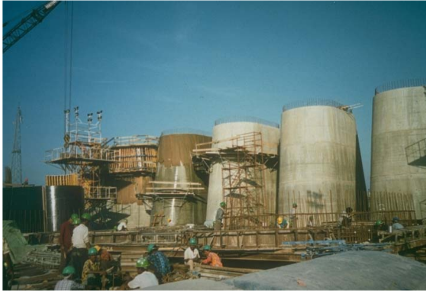
Figure 3.24. Precast Pile Cap Shells (Jamuna River Bridge)
