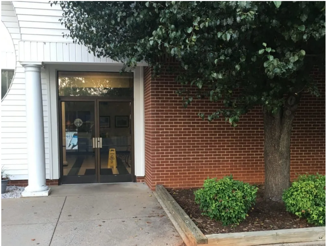
Rutherford County government administration building houses the county government in Rutherfordton. Ben Ledbetter / Carolina Public Press
