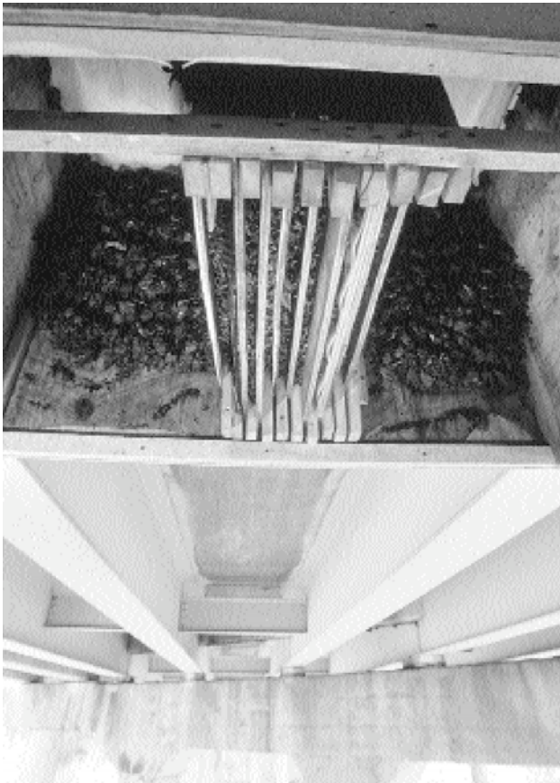
Figure 20. Several designs of the Texas Bat-Abode, such as this one modified for a steel I-beam bridge, have been used to attract thousands of bats.
