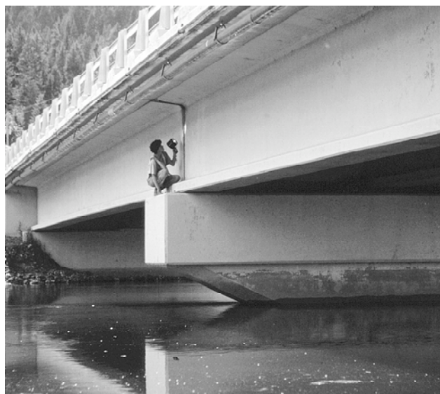
Figure 6. This Idaho bridge sheltered a nursery colony of several hundred little brown myotis, the northernmost colony discovered during the survey.
