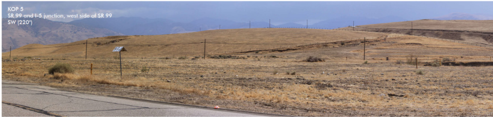
Figure 4.1-4: Photo Locations, Existing Views for Key Observation Points 5 and 6
