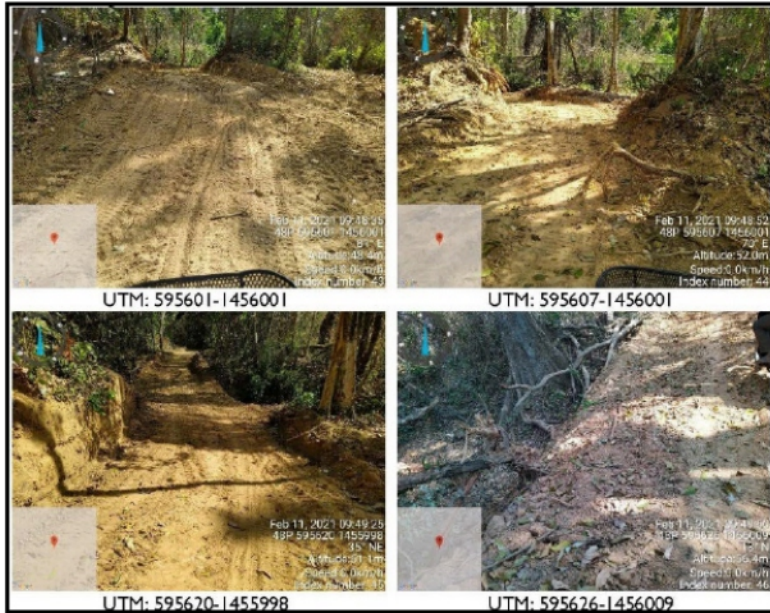
Figure 4 New logging roads constructed inside Prey Lang documented in February 2021.
