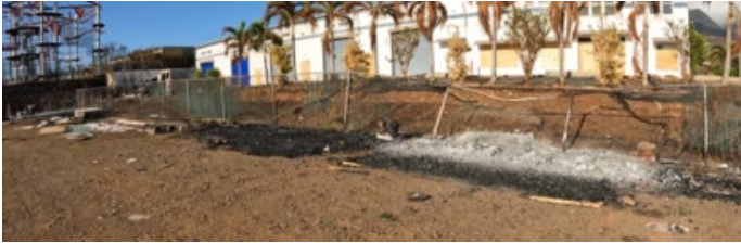
Figure 4.3.5.1.14 Materials storage area burned by embers (1 █ Kupuohi Street).
