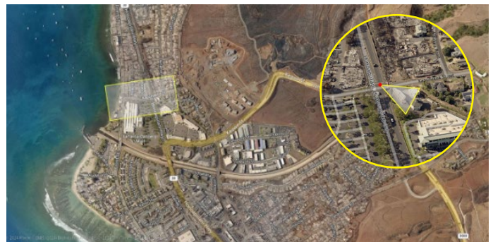
Figure 3.8.2.1 Several downed utility poles and powerlines in the northbound lane of Hwy-30 and Kapunakea Street. Photo taken August 8, 2023, at 16:52. Inset: Viewpoint of photo of downed utility poles and electrical lines at Hwy-30 and Kapunakea Street.
