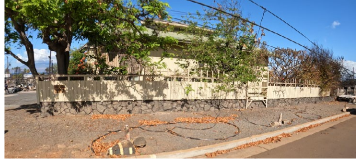
Figure 4.3.5.2.14 12█ 'Ainakea Road (Front view, oriented west).
