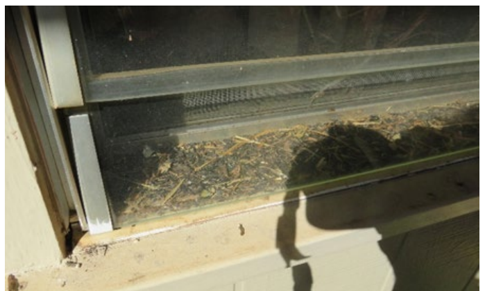
Figure 4.3.4.4.14 Louvered windows left partially ajar where debris collected, including charred remains of possible embers. An intact screen behind this window kept these materials from entering the structure and possibly igniting interior contents.
