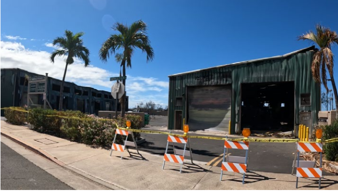
Figure 4.3.5.1.20 Emerald Plaza Building A consumed by fire.
