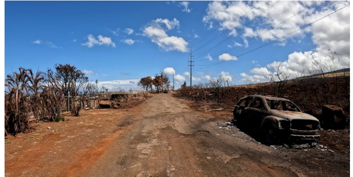
Figure 4.3.5.2.6 Car located at edge of construction site that supported the fire jumping Oil Road from the east-mauka (right to left).
