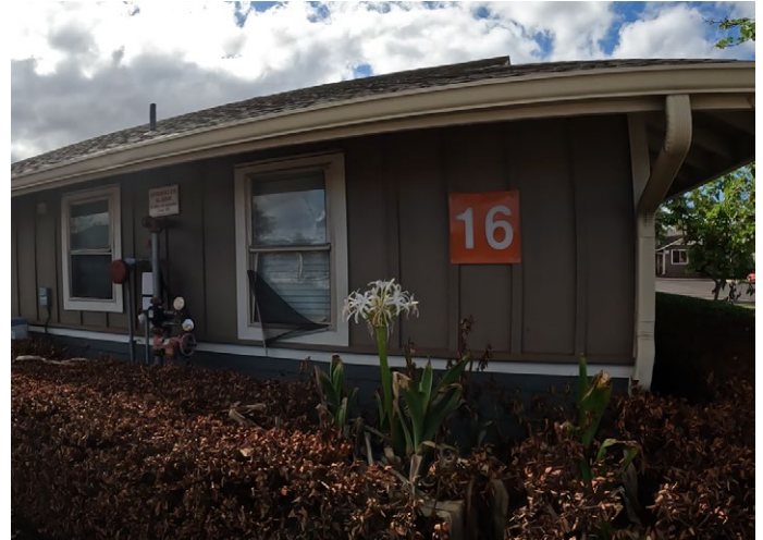
Figure 4.3.3.4.11 Thermal damage (window) to the front of Building 16, across from Building 15 (destroyed).
