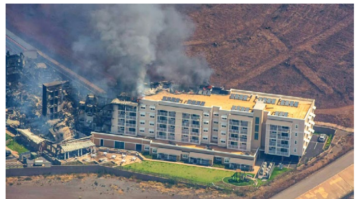
Figure 4.3.5.1.24 Kaiāulu o Kupuohi Apartment complex continuing to burn following the August 8, 2023, fire. 261
