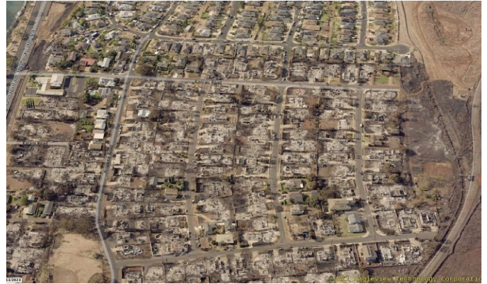
Figure 4.3.5.3.1 Aerial imagery of the North Zone, between Kaniau Road and 'Aipuni Street, which is the most northern area of Lahaina affected by the August 2023 Maui fires.
