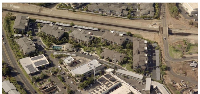
Figure 4.3.3.4.1 Pre-fire aerial imagery (captured August 10, 2021) of Opukea Apartments.
