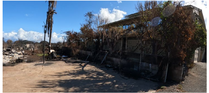
Figure 4.3.5.2.16 12█ 'Ainakea Road (rear view, oriented northeast).
