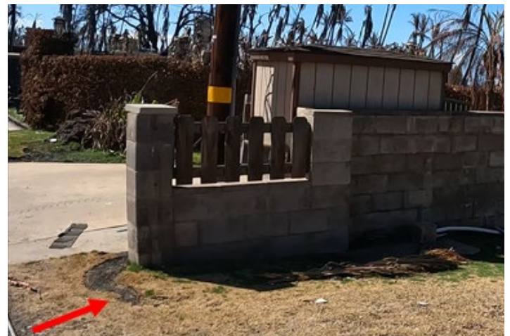
Figure 4.3.4.3.4 Tall, lush vegetation was planted along block walls on either side of the driveway to 3█ Front Street, which may have provided protection to the 3█ and 3█ Front Street lots. The block wall south of 385 Front Street also influenced the ember movement. Note pile up in corner of wall (bottom left) and wind driven burn scar in grass around the wall toward the front of the structure showing the likely path of ground based embers deflected towards the north and away from the open garage (bottom right).
