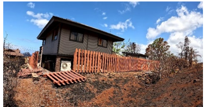
Figure 4.3.5.3.5 The surviving accessory structure at 16███ Lokia Street was near the eastern (mauka) property line, but was buffered from the grassland by a garden (note intact hoses and stone landscaping separating from the grass) and a fence. The structure was elevated such that the damaged windows were a longer distance from the burning vegetation than a single-story structure. Charred sections of fence were broken away from the posts and burning was stopped. Broken windows were boarded up from the inside by the time images were collected.
