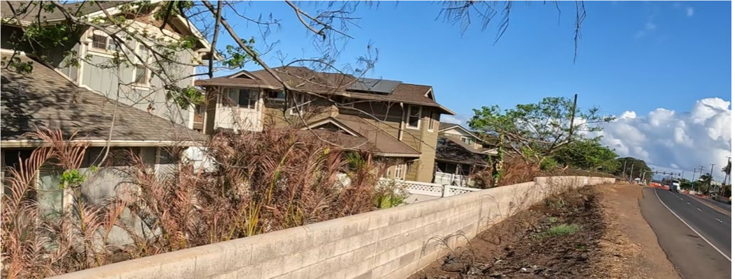
Figure 4.3.3.5.3 Concrete barrier wall along Hwy-30.
