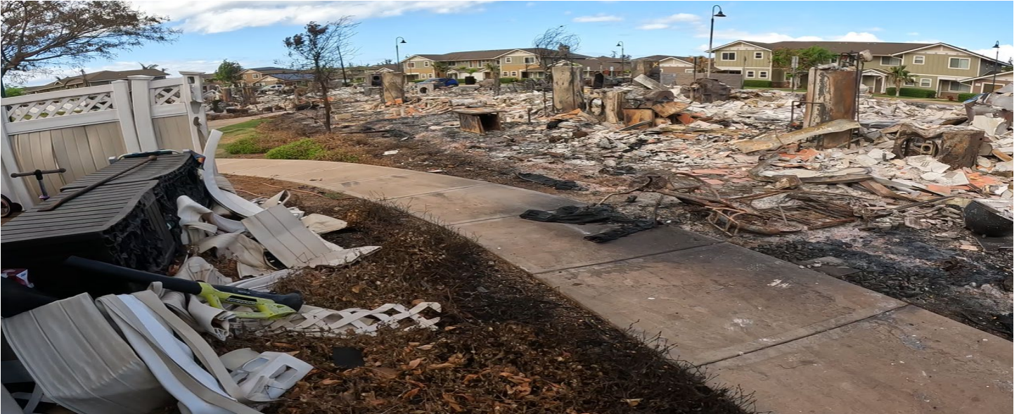
Figure 4.3.3.5.9 Ground-based photograph of space between Building 13 (shown on the left of the image) and Building 14 (shown on the right).
