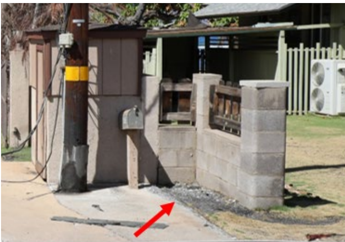
Figure 4.3.4.3.4 Tall, lush vegetation was planted along block walls on either side of the driveway to 3█ Front Street, which may have provided protection to the 3█ and 3█ Front Street lots. The block wall south of 385 Front Street also influenced the ember movement. Note pile up in corner of wall (bottom left) and wind driven burn scar in grass around the wall toward the front of the structure showing the likely path of ground based embers deflected towards the north and away from the open garage (bottom right).
