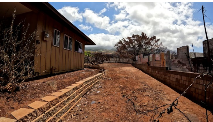
Figure 4.3.5.3.6 The 16 Lokia Street structure did not appear damaged by the grass fire to the east (mauka) sides (top left) or destroyed structure west (makai) of Lokia Street (top right). The structure was heavily damaged from radiant heating from the destroyed structure to the south (bottom left) and north (bottom, right).
