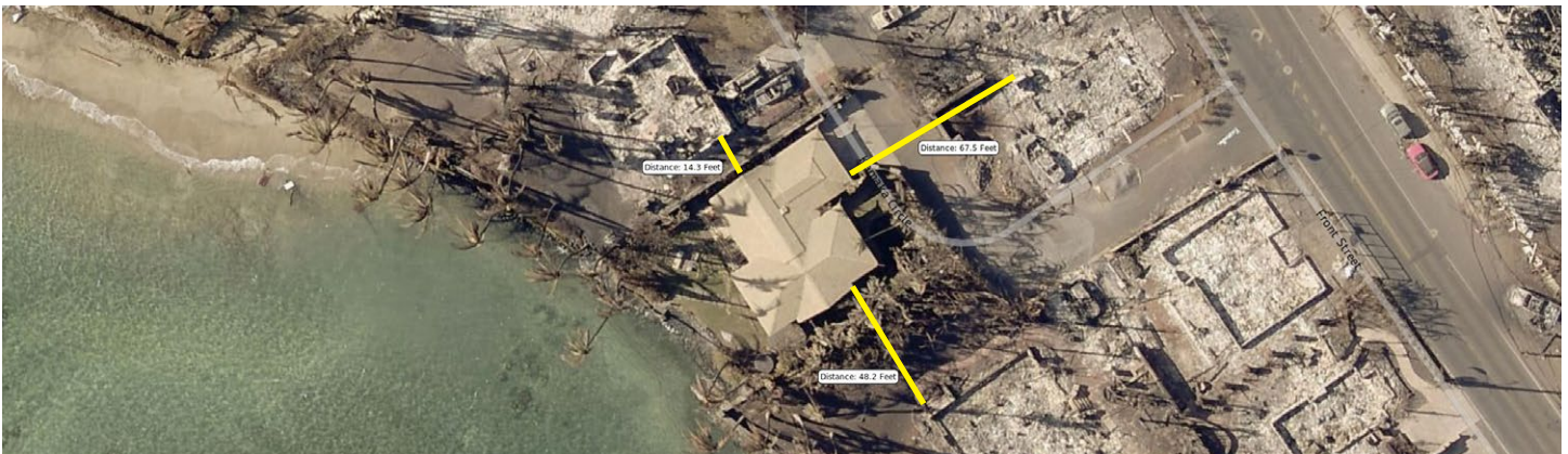
Figure 4.3.3.6.7 Post-fire aerial imagery of 1 Kamaka Circle (damaged), surrounded by destroyed structures.
