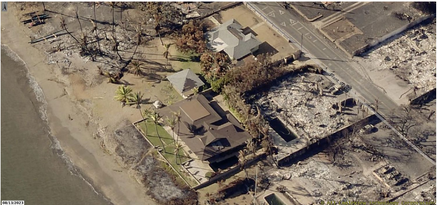
Figure 4.3.4.2.20 Examples of open/broken windows and/or screens in this cluster of surviving homes. (Figure 4.3.4.3.1 continues on page 254.)
