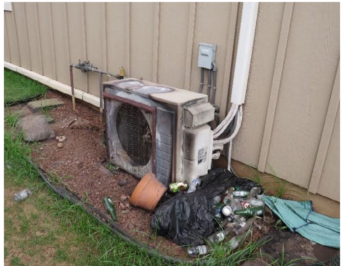
Figure 4.3.3.3.4 Isolated fire damage to 311 Komo Mai Street. Spot fire (ember ignition) caused localized damage, but did not spread to the structure, likely due to defensive actions.
