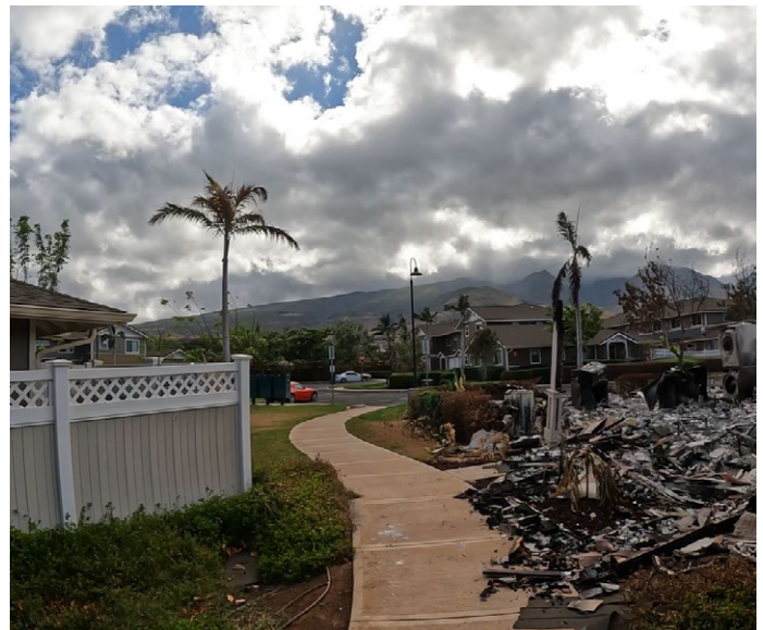
Figure 4.3.3.5.10 Photograph of space between Building 12 (shown on the right of the image) and Building 13 (shown on the left), showing minimal damage to the vinyl fence.
