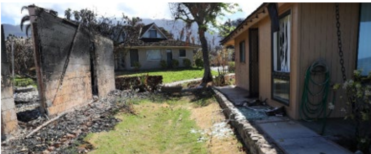
Figure 4.3.4.4.8 Damage to the north end of 4 Pualoke Place immediately adjacent to the destroyed structure at 3 Pualoke Place. A tree to the east (mauka) of the structure sustained deep charring, likely from embers gathering in cracks, fissures, or scars in the tree bark (top left). Window damage on the north structure wall (top right) ranges from single pane cracking to vinyl frame warping (middle left) to complete pane fallout (middle center). Plastic vent cover and gutters melted and fell. Paint bubbled and peeled across most of the surface. No apparent indication of charring or damage to wood shake roofing materials or wood wall substrate (top right and middle right). Grass remained green between the destroyed and damaged structure. Garden hose noted at the corner of the structure (bottom left). Inset: Viewpoint showing area shown in the photographs above.
