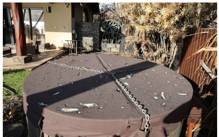
Figure 4.3.3.6.10 Ember damage of a hot tub cover reveals the noticeable size variation of embers encountered during the fire.
