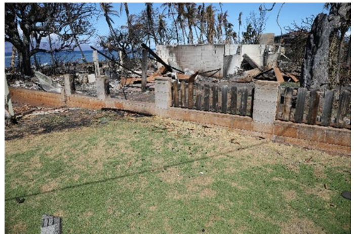
Figure 4.3.4.3.7 Burnt, charred, and broken wooden fence from the 3-3 Front Street property line directly connected to the structure at 3 Front Street. Wooden fences can act as a “wick,” carrying fire from one structure to the next. The northernmost panel was disconnected from the rest of the fence, removing this mechanism of fire spread.
