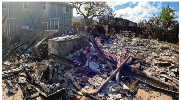
Figure 4.3.3.5.4 Destroyed single family home at 2█ Kahoma Village Loop from the front (north).
