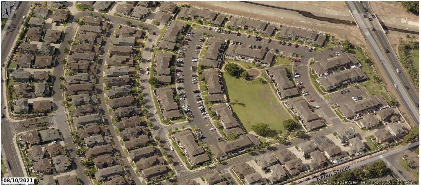
Figure 4.3.3.5.1 Pre-fire aerial imagery (captured August 10, 2021) of Kahoma Village before the fire.
