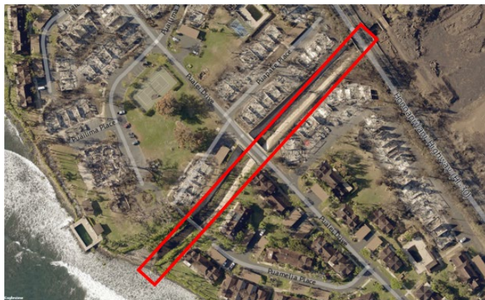
Figure 4.3.4.4.9 Kaua'ula Stream running through Puamana provided a physical separation between the northern section (where structures were destroyed between Hwy-30 and the coast) and the rest of the community (where destroyed structures were limited to the area between Hwy-30 and Pualei Drive).
