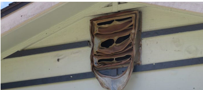
Figure 4.3.4.2.18 Radiant heat damage to the structure and household belongings at 447 'Āli'ō Street was noted primarily on the north side.
