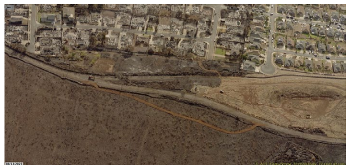
Figure 4.3.5.3.3 Fire in the grassland along the eastern edge (mauka) of the northern zone crossed over Oil Road to the eastern edge (mauka) of properties on Lokia Street and Kaniau Road. The north flank vegetation fire remained east (mauka) of Oil Road between 'Aipuni Street and Leialii Parkway, after which the fire moved back west (makai). Note: North is to the right on these images.
