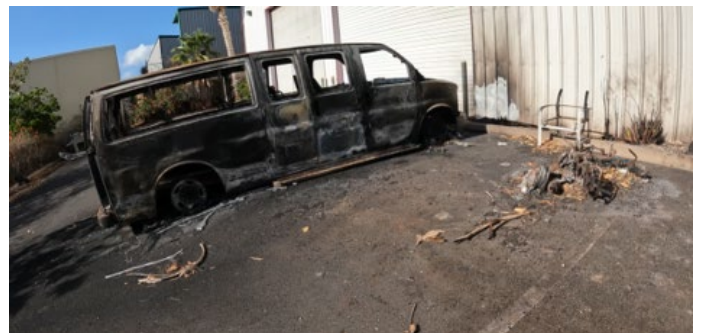
Figure 4.3.5.1.19 Van consumed by fire with thermal damage to 1 █ Kupuohi Street.
