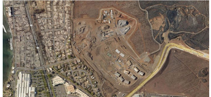
Figure 4.3.5.2.1 Post-fire aerial imagery of the Keawe Street Apartments at the Villages of Leialii construction site and surrounding neighborhood.
