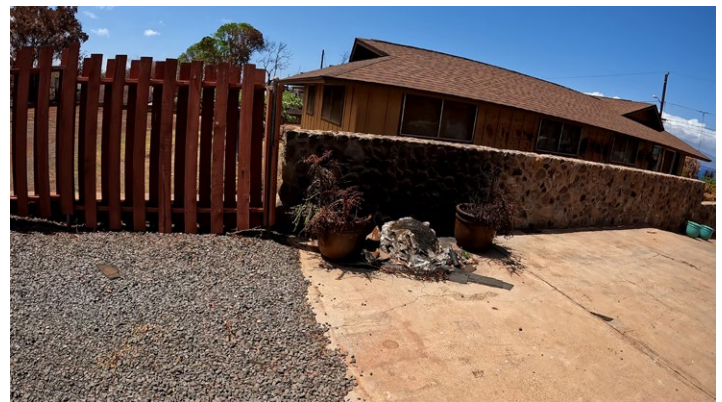
Figure 4.3.5.3.6 The 16 Lokia Street structure did not appear damaged by the grass fire to the east (mauka) sides (top left) or destroyed structure west (makai) of Lokia Street (top right). The structure was heavily damaged from radiant heating from the destroyed structure to the south (bottom left) and north (bottom, right).
