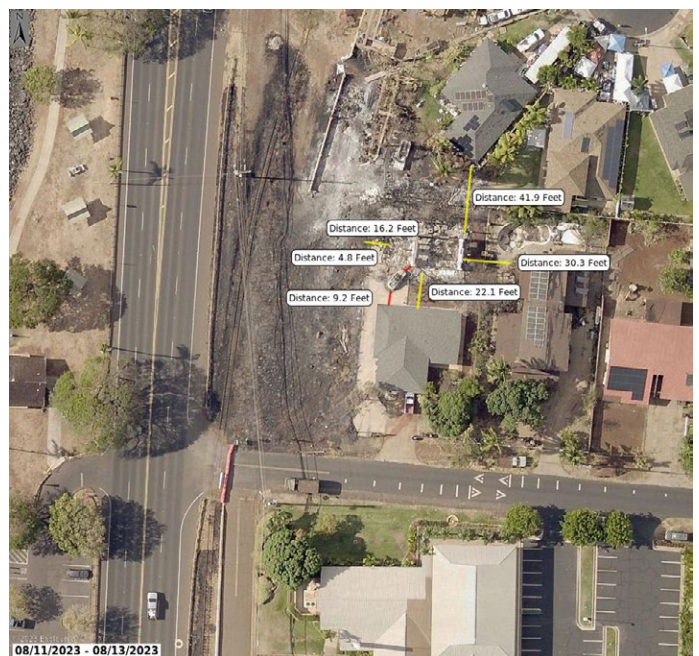
Figure 4.3.5.3.8 Structure spacing near destroyed accessory structure at 1█ Kaniau Street.
