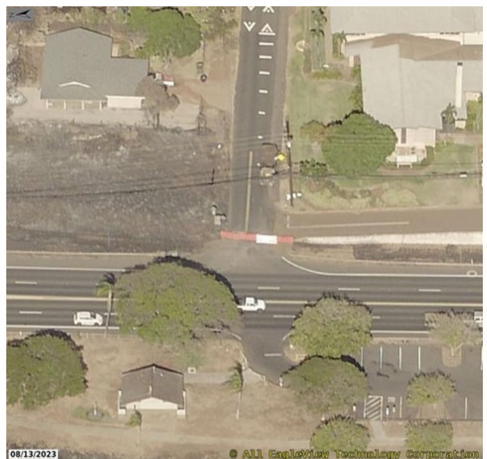
Figure 4.3.5.3.9 Tall dry grasses are noted on the northeast corner of Kaniau Road and Hwy-30 in August 2020 (top), which could have provided a receptive fuel bed for fires along the railroad tracks or embers moving down (makai) Kaniau Road to ignite these grasses in August 2023 and travel to structures in the immediate vicinity (bottom). Note: North is to the left of these images.
