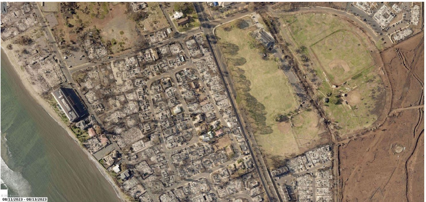
Figure 4.3.4.1.1 EagleView image of the 400 block of Front Street showing the survival of six (6) primary structures on the west (makai) side of the street.
