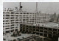
Completed new DA building in Kasumigaseki, Tokyo (From Etchujima to Kasumigaseki)
