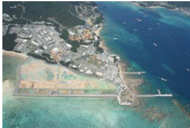
Progress of landfill work (April 2024)
