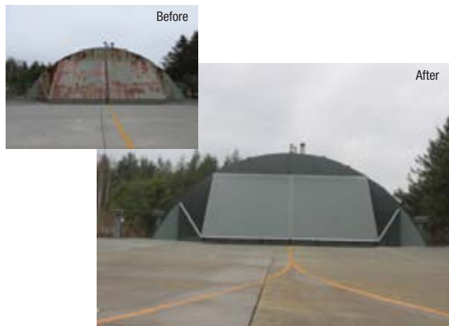
An improved aircraft shelter for F-15 fighters at the ASDF Chitose Air Base
