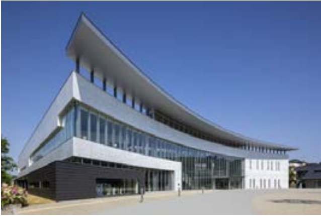
“Sakaiminato Citizens Exchange Center (Minato Terrace)” established as part of an urban development support project (Sakaiminato City, Tottori Prefecture)
