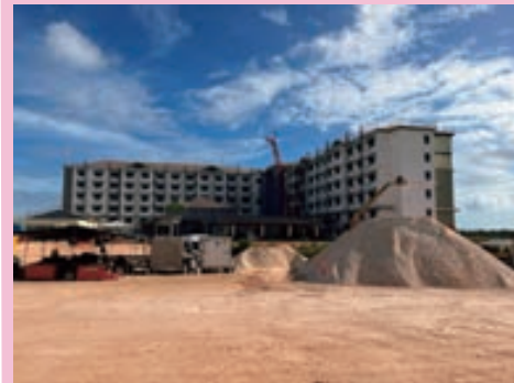
Construction of facilities in Finegayan
