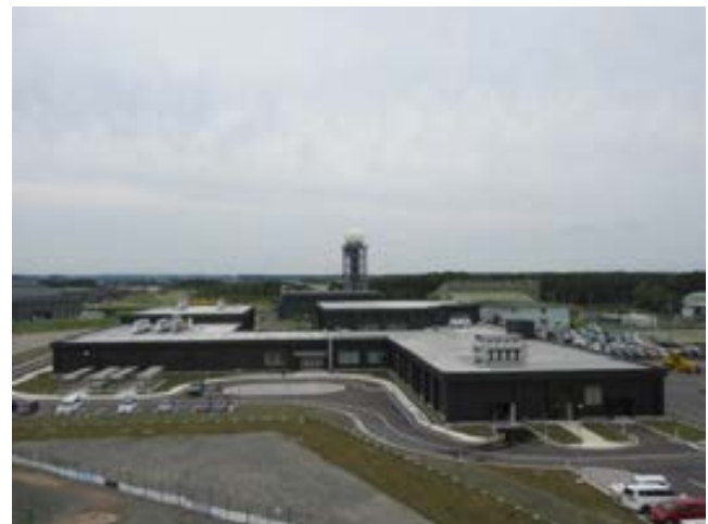
Facilities for receiving F-35A and F-35B fighters (image)
