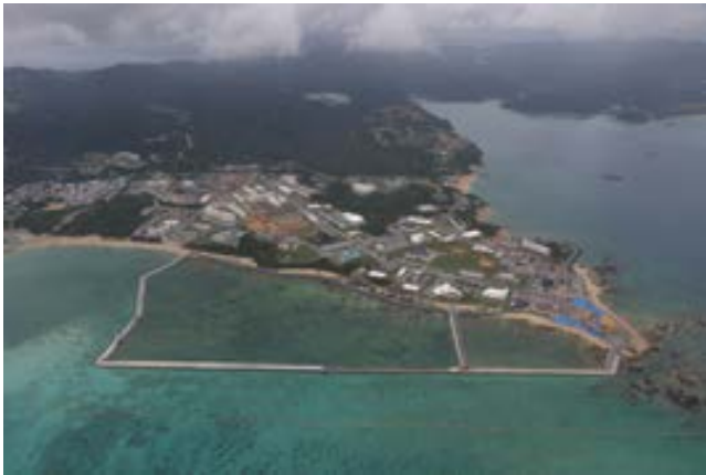
Progress of landfill work (November 2018)
