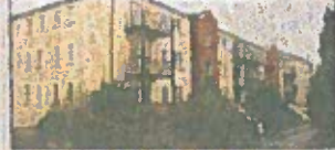
The Skyscraper at home of construction in the city
