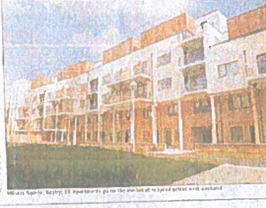
Santry, Dublin 10, is a large apartment complex with a glass facade.
