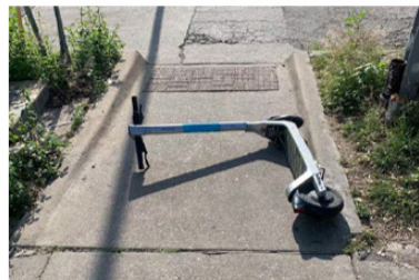
Blocking ADA ramp
