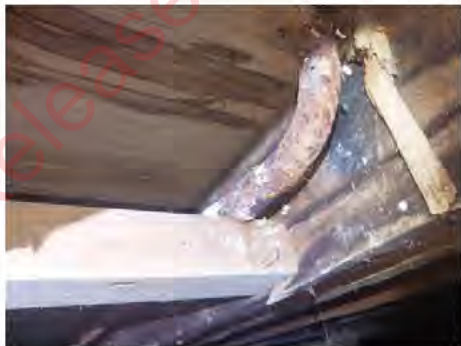
Image shows highly contaminated crawl space. Thermal insulation on the floor. In this condition the likelihood that the sub-contractors would have needed to crawl through this is probable.
