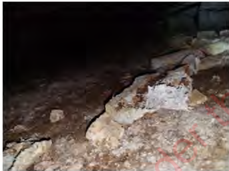
Image shows highly contaminated crawl space. Thermal insulation on the floor. In this condition the likelihood that the sub-contractors would have needed to crawl through this is probable.
