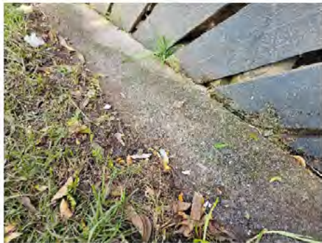
Image shows ACM still present after the clearance certificate has been issued..
