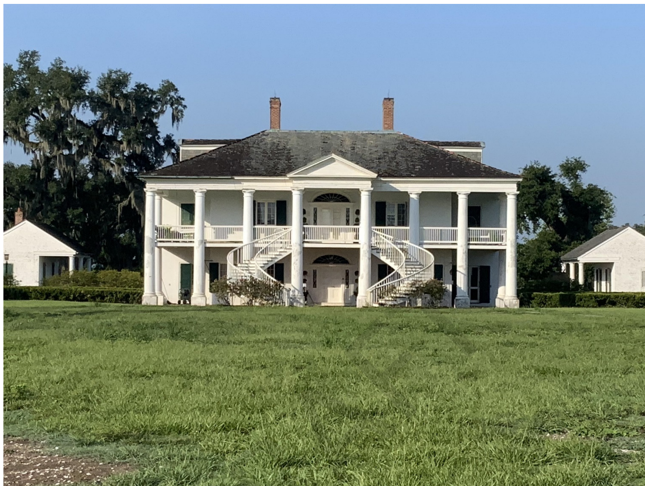
1 2 3 4 Figure 3-49. Photo of the Evergreen Plantation, located at 4677 HWY 18 in Wallace (ID# 481, PIDN 0300027410). Source: HHM , August 2023, https://data.hhminc.com/place/143557 .
