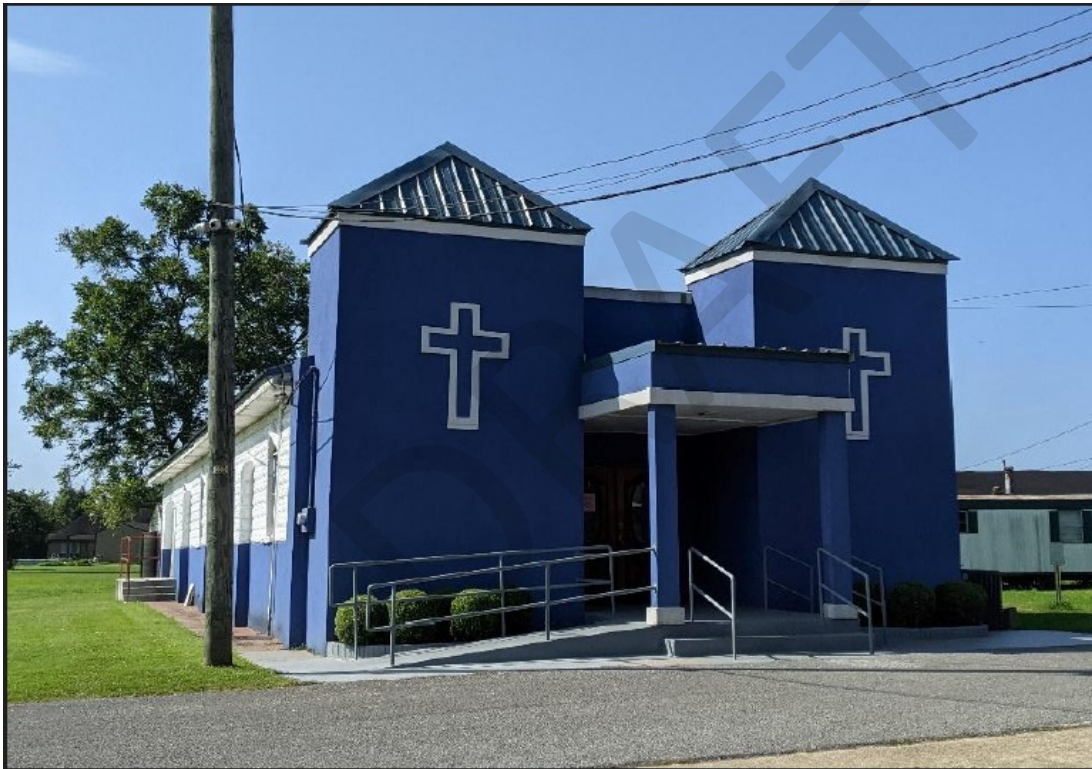
Figure 2-14. View of Woodville Baptist Church.
