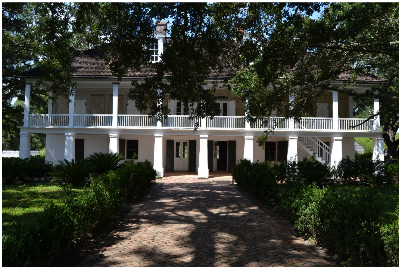
1 2 3 4 Figure 3-48, Photo of the Whitney Plantation, located at 5099 HWY 18 in Wallace (ID# 440, PIDN 0300069311). Source: HHM, August 2023, https://data.hhminc.com/place/143555/images .
