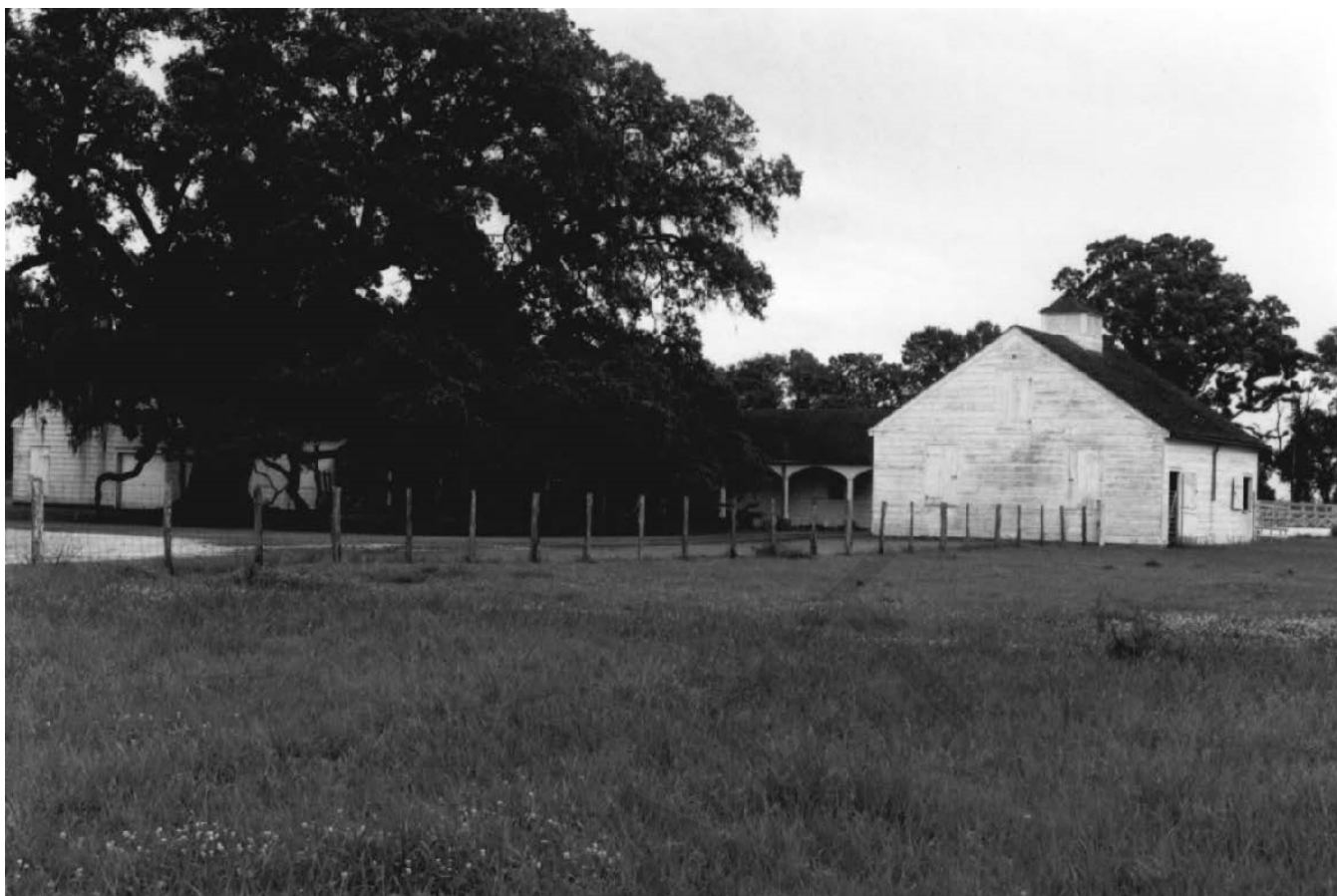
1 2 Figure 3-45. Photo of the stable at Evergreen Plantation. Source: Fricker, Donna. "Evergreen Plantation." National Register of 3 Historic Places Nomination. May 1991. 4
