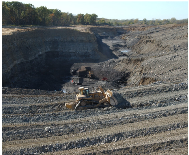
ILLINOIS Former coal mine site undergoing reclamation. © Tami Heilemann
