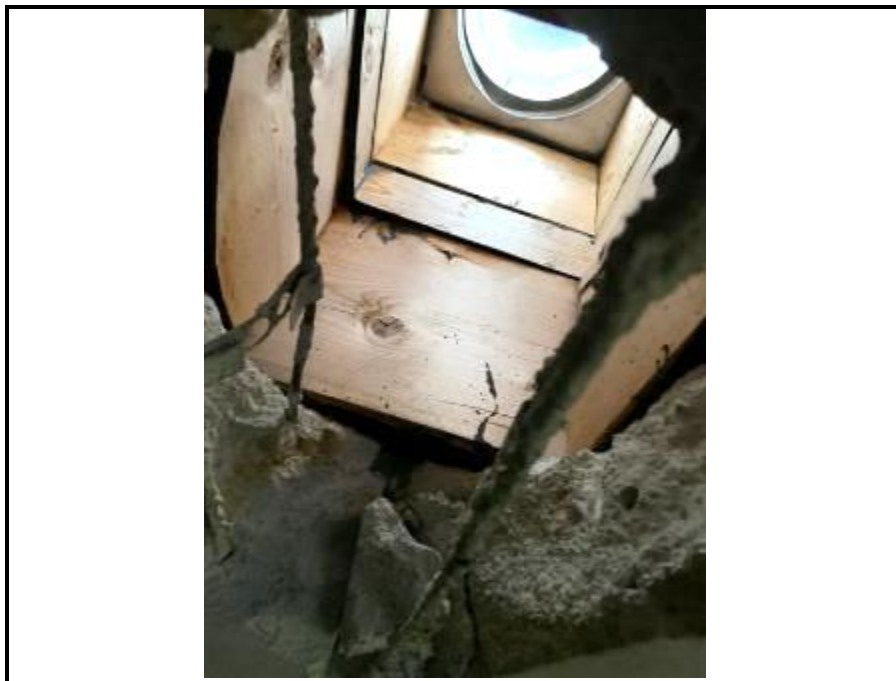
Photograph 4 Repair Location A1.4 – Unreinforced field modification
