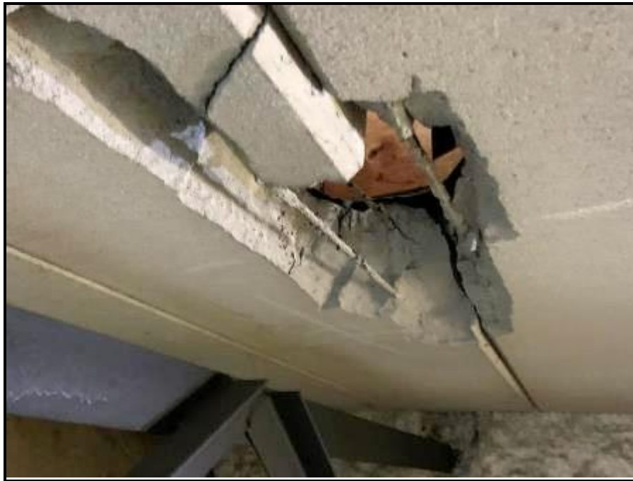
Photograph 3 Repair Location A1.2 – Unreinforced field modification
