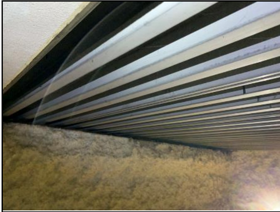
Photograph 1 Roof Area A1 – RAAC replacement with steel deck
