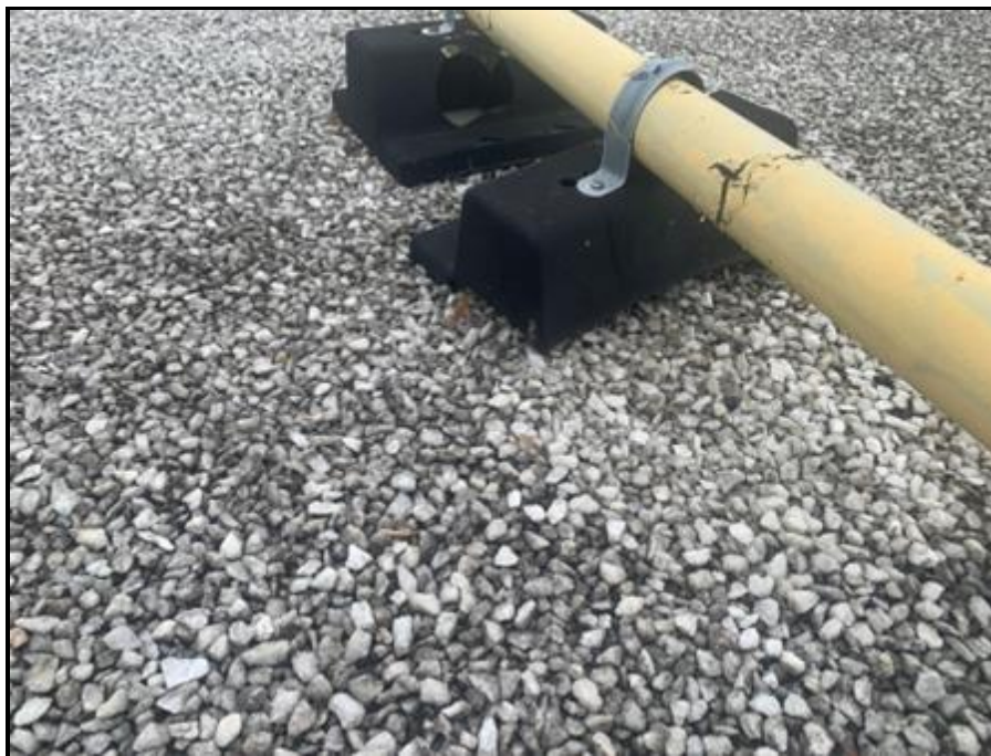
Photograph 22 Repair Area A2 - Repair broken gas line support
