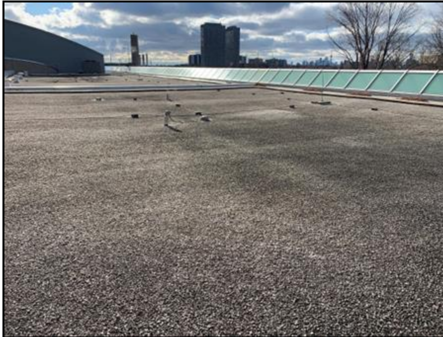
Photograph 34 Repair Area A5 - Remove minor accumulation of organic debris at roof drain located on the north end of roof area A5
