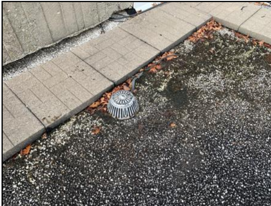
Photograph 34 Repair Area A5 - Remove minor accumulation of organic debris at roof drain located on the north end of roof area A5
