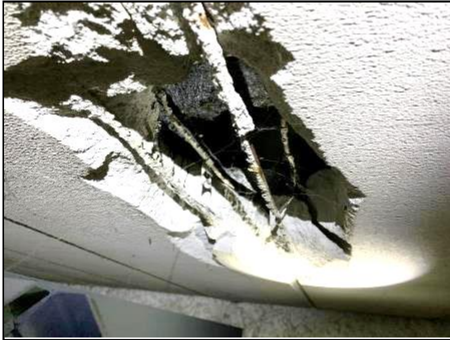
Photograph 5 Repair Location A1.5 – Unreinforced field modification
