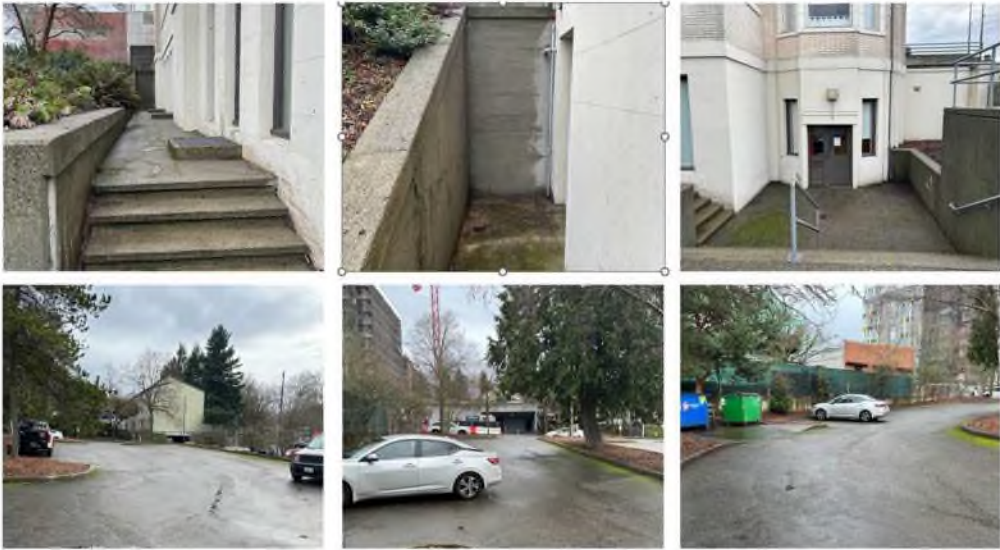
• Blowing and removing crack weeds at Medgar Evers Swimming pool
