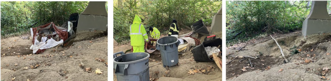
NE 50 th St Off-Ramp
