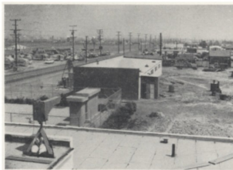
Fig. 7 - Transmissometer sending and receiving equipment at Dominguez aerometric station. Receiver is in lower left-hand corner; light source is bright spot on lower right-hand corner of roof in middle distance
