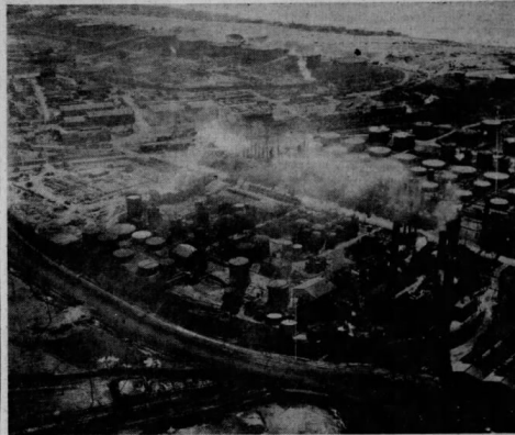
WHAT ABOUT IT? —Oil refineries in Los Angeles area undoubtedly contribute to smog nuisance. The industry is striving for a solution but fast technological changes in gasoline processing make radical revisions difficult. Here is El Segundo plant.
