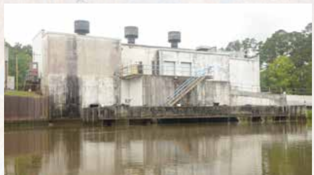
The City of Savannah's water intake on Abercorn Creek was built in 1948. Since then it has played an oversized role in the growth and sustainability of the region. The surface water source has been especially important as limits on groundwater withdrawals have been put in place because of saltwater intrusion.
