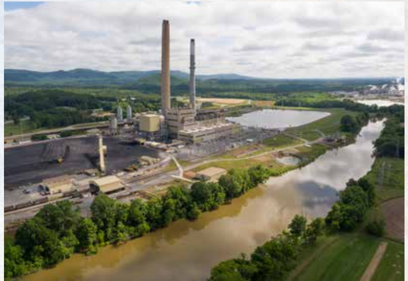
Located on the Coosa River west of Rome, the now shuttered Plant Hammond, a coal-fired power plant, was home to four coal ash ponds. Ash in three of those ponds is slated to be dewatered and moved off site to lined landfills. A final ash pond has been capped in place. That pond holds some one million tons of coal ash that is in contact with groundwater.
