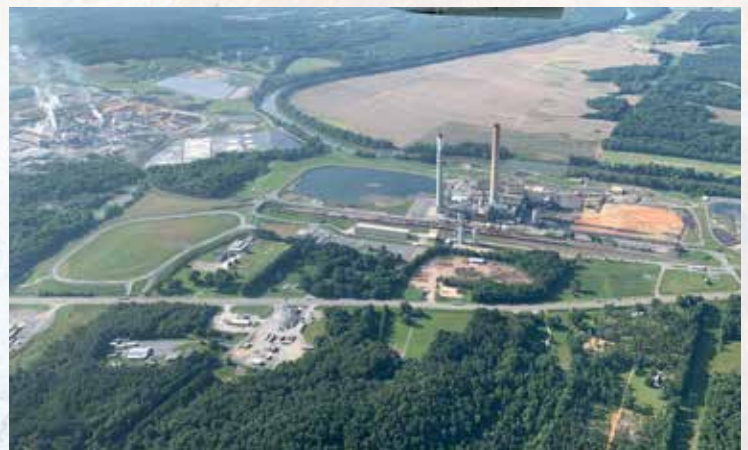
Located in the far left of this photo, Ash Pond 3 now appears as a 25-acre grassy mound along Ga. 20 in the foreground. It looms over Pisgah Baptist Church to the west and Cabin Creek to the east. It appears benign, but in fact, beneath the surface coal ash extends some 44-feet deep and ten feet below the upper limit of the groundwater table.
