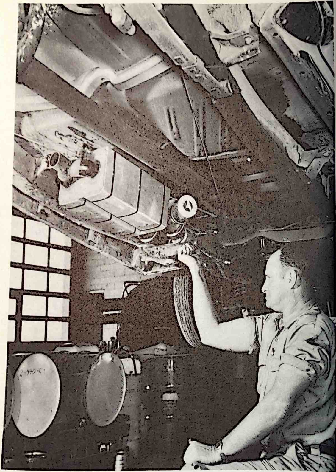
CHAPTER IV - FIG. 4 Houdry catalytic muffler being installed on automobile—Southwest Research Institute
